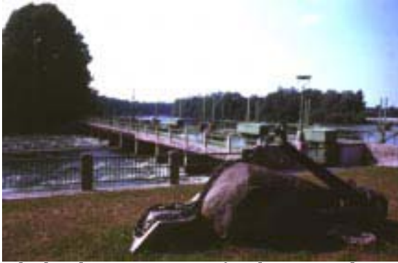
The head gate structure for the 1972 Olympics near Munich, Germany.
