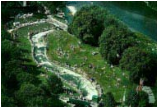
Aerial view of finish area. The return spillway to the Lech River is in the top center of the picture.
