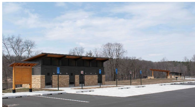
New restrooms and picnic shelter in day use area.
