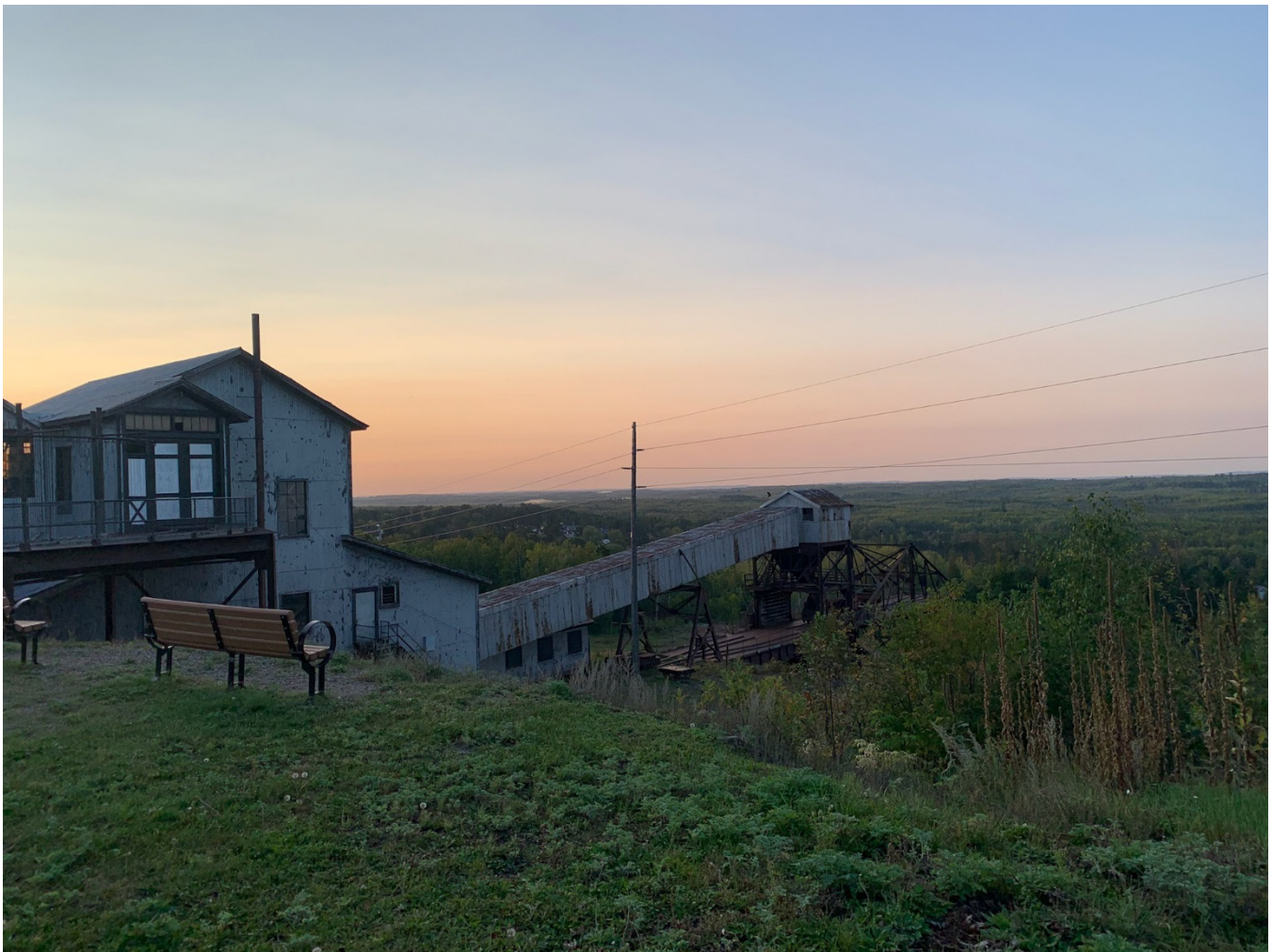
Lake Vermilion-Soudan Underground Mine: Crusher house. - Jim Devries
