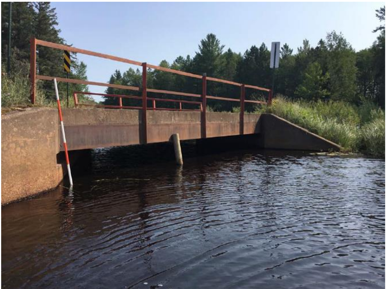
Figure 12. Current Net River Forest Road Bridge, undersized for water crossing.
