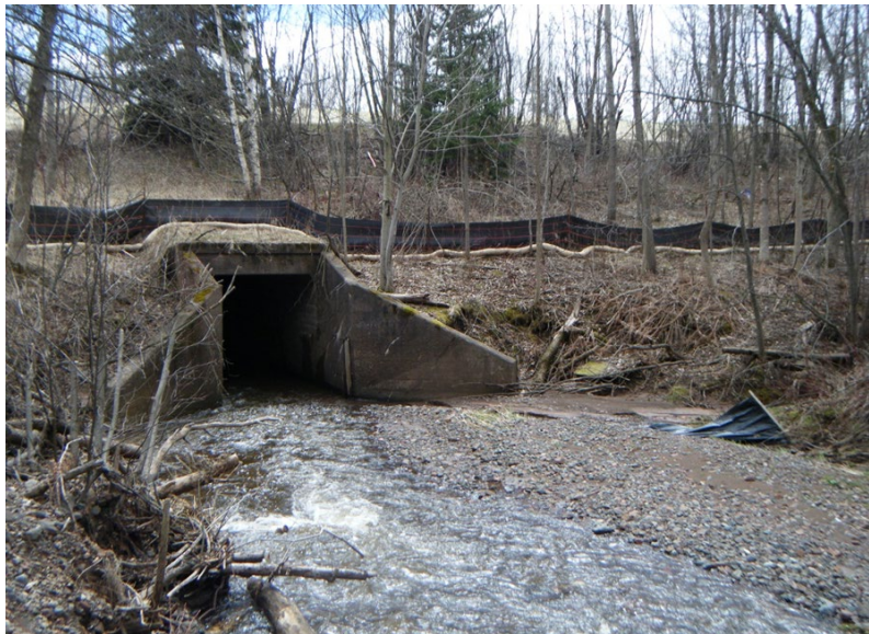
Figure 33. Lower Knowlton Creek culvert under the Munger Trail.
