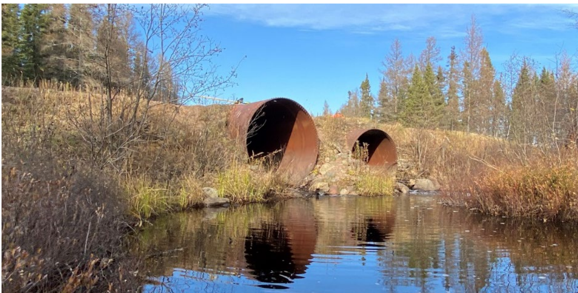
Figure 38. West Branch of the Baptism Culvert.
