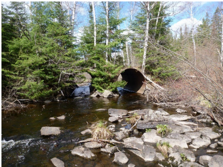
Figure 34. Ramstad/Moosewalk culvert before replacement with a bridge.
