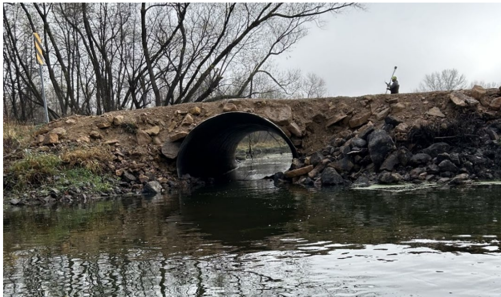
Figure 29. Gorman Lake Culvert on Dodd Road, downstream of Gorman Lake Outlet.
