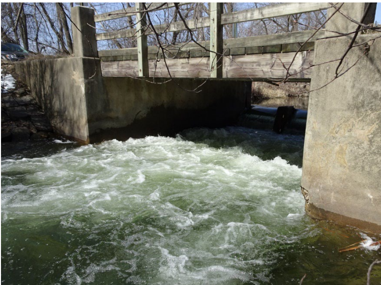
Figure 31. Lake Calhoun Bypass Dam.
