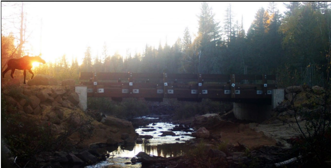
Figure 37. Moose walks over the new bridge at sunset.
