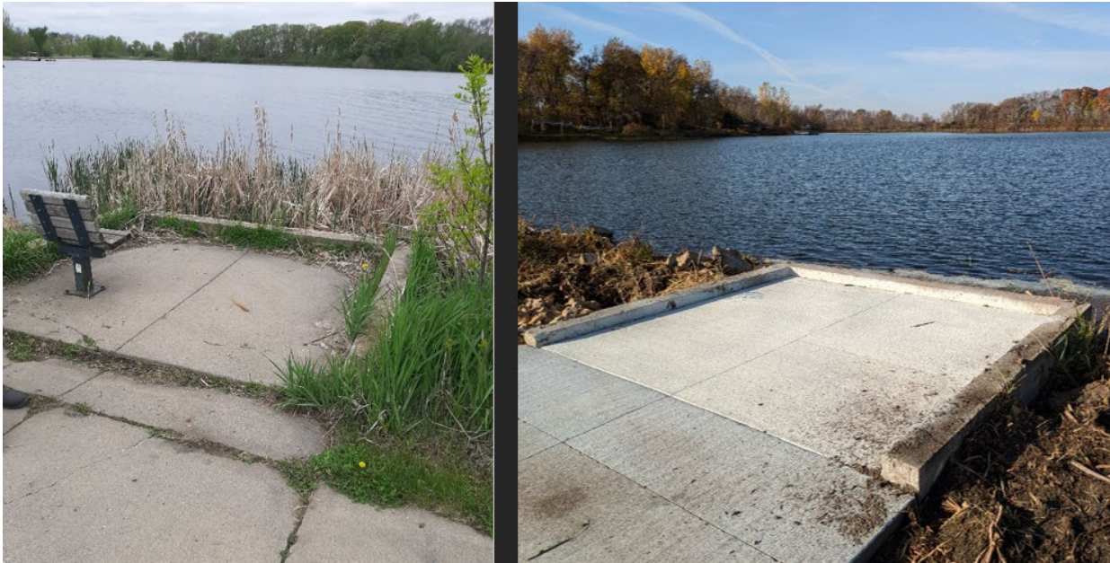
Figure 18. Before (left) and after (right) photos of a shore fishing station at Buckmaster Bridge.
