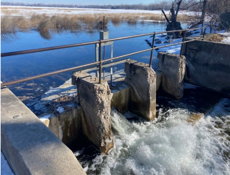
Figure 30. Lake Calhoun Outlet Dam.
