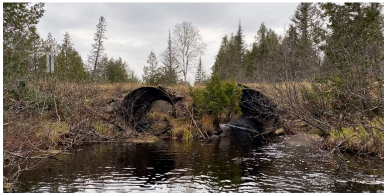
Figure 39. Manitou River Culvert.
