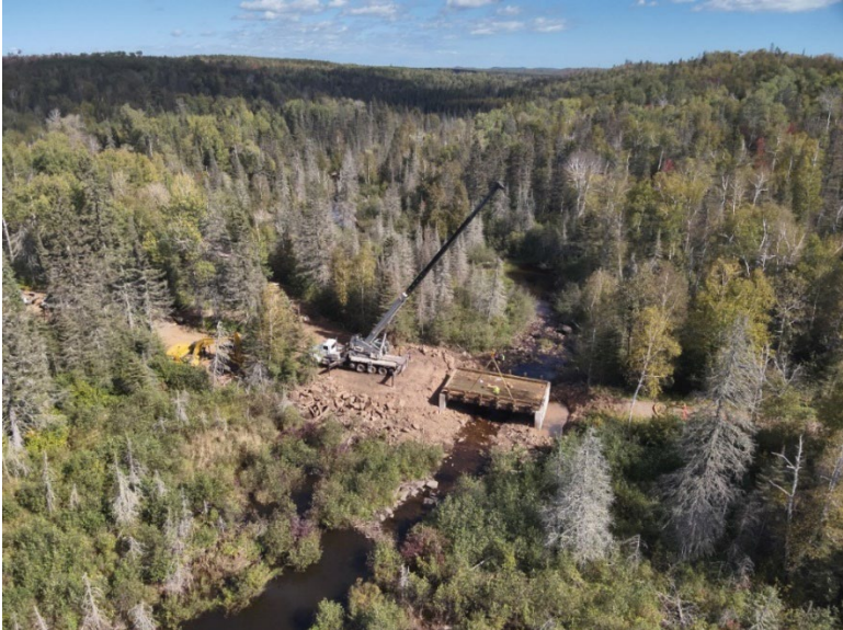
Figure 36. Ramstad/Moosewalk snowmobile trail bridge just after construction. The stream channel is now passable by fish and the bridge is wide enough to sustain larger floods.
