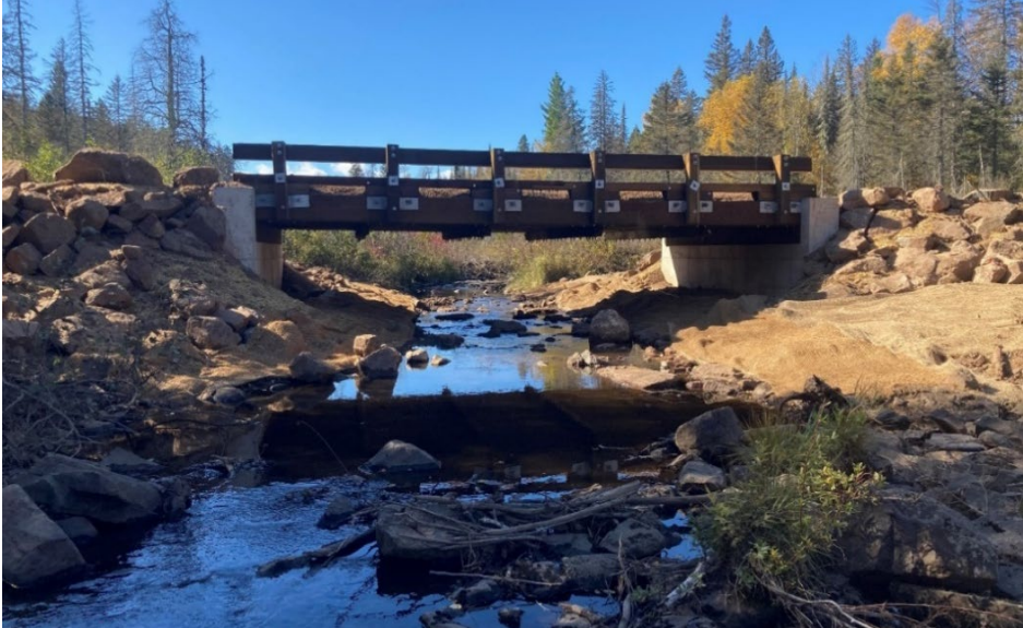
Figure 36. Ramstad/Moosewalk snowmobile trail bridge just after construction. The stream channel is now passable by fish and the bridge is wide enough to sustain larger floods.
