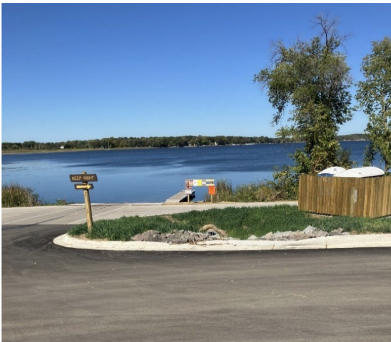
Figure 13. Sugar Lake (South) PWA after improvements to the ramp and parking lot.
