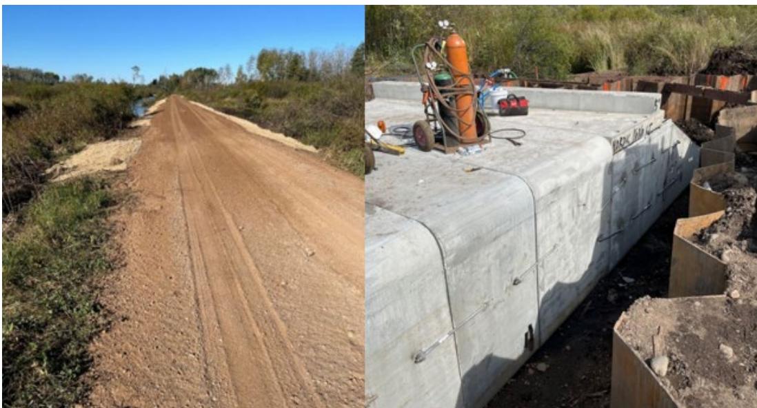
Figure 9. Construction photos of Ditchbank State Forest Road.
