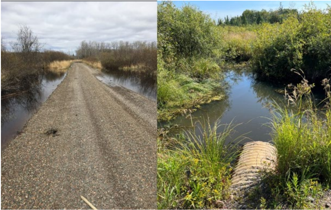
Figure 8. Preconstruction condition of Ditchbank State Forest road.
