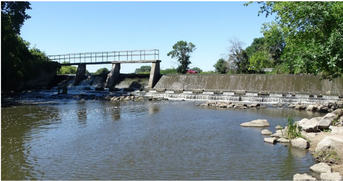
Figure 26. Crissy Lake Dam.
