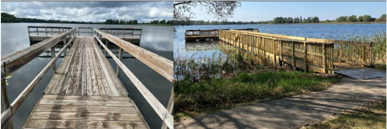
Figure 16. Bass Lake Fishing pier, before (left) and after (right).
