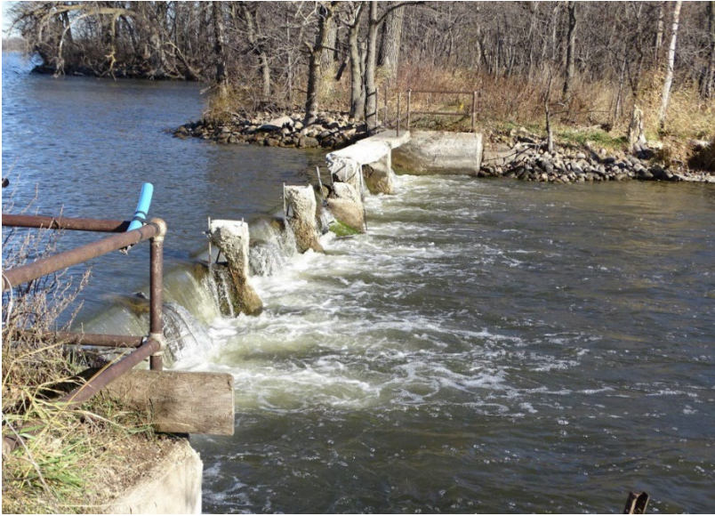
Figure 24. Perkins Lake Outlet Dam.
