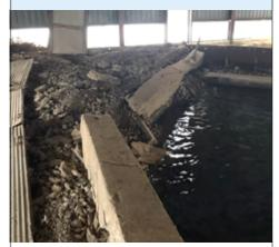
The crumbling spring pool wall (shown above) at Lanesboro Hatchery and the failing pond dike at Waterville Hatchery (shown below) are just two examples of aging infrastructure that threaten production of millions of walleye, muskellunge, and trout across the state's hatchery system.
