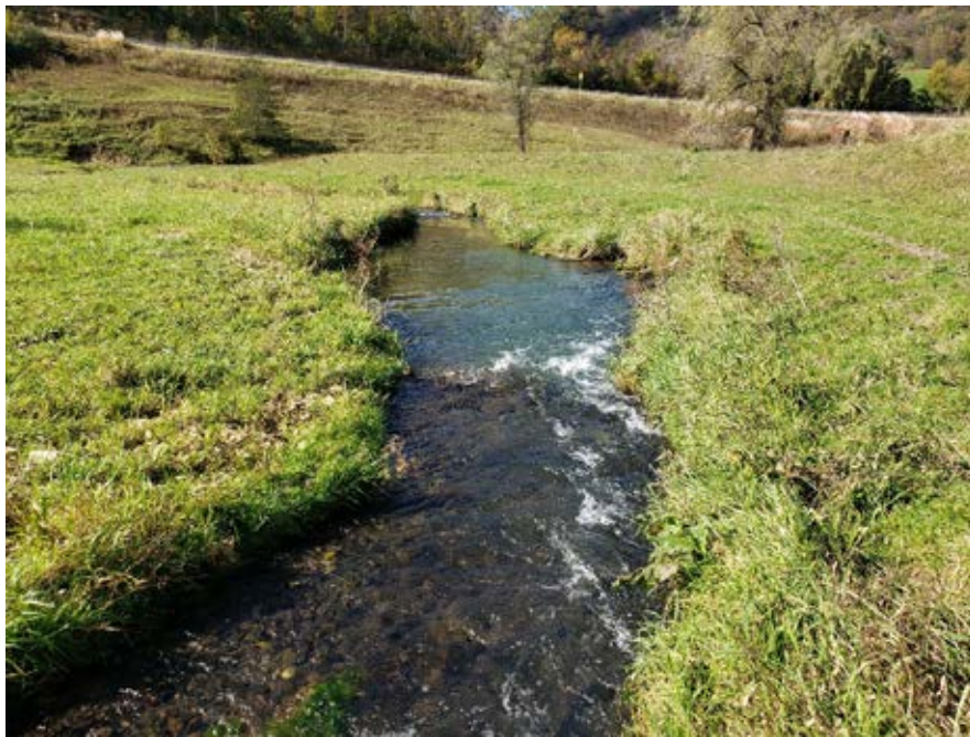
Photo 22-1. Example of Pickwick Creek eight years after construction. Much of the stone toe used to line the channel is overgrown with vegetation. Low banks help to support the stability of the stream. Photo taken 10/17/19 by Mark Prancus, Cardno.
