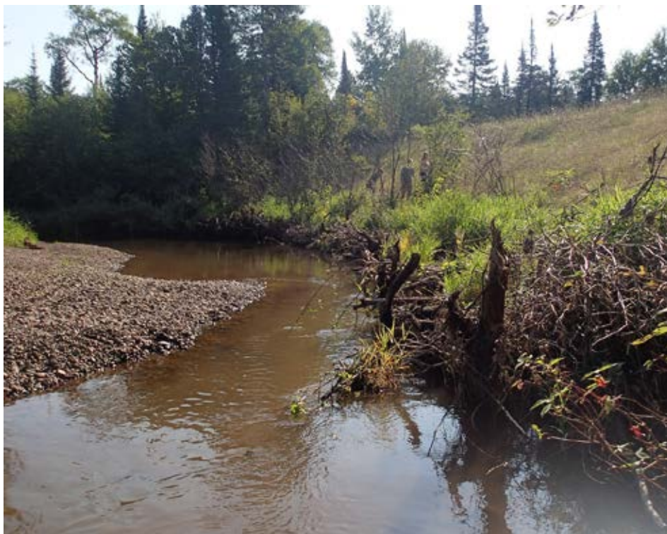
Photo 4-8 Toewood rootwads and first year's vegetation growth on slope. Facing upstream during low water conditions. Site visit 08/24/2012.
