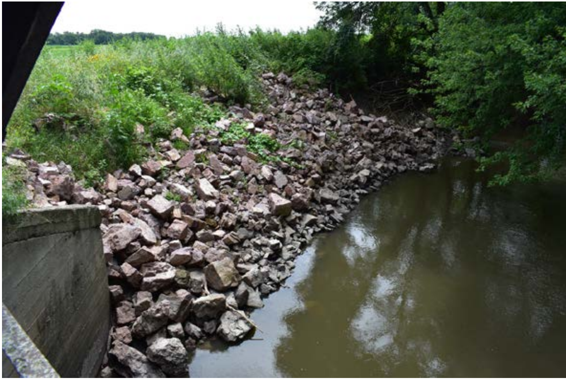
Photo 2-5 View of Adams near Bridge. Riprap protection bank. Photo taken by Ed Matthiesen during site visit (8/13/19).
