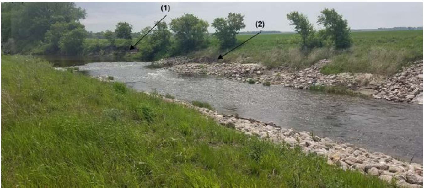
Photo 16-11 Sand Hill River fishway ramp #4 after the original drop structure was modified for fish passage. Upstream of the project area a washout is visible (1). Washout area will be repaired after the culvert connecting the reach to a side channel is addressed. There are also limited bare spots that could be reseeded in the project area (2). Photo taken by Ed Matthiesen during site visit (6/4/2019).
