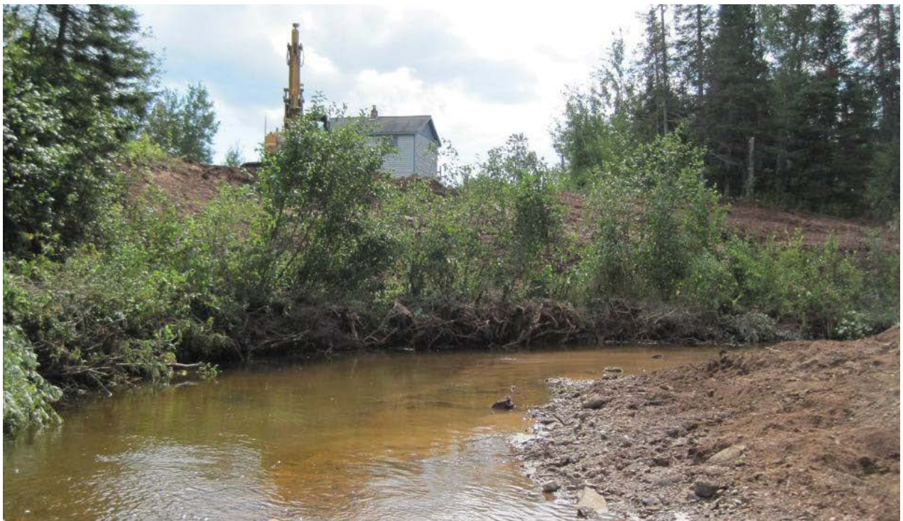
Photo 4-6 Toewood completed 09/13/2011. Top layer of toewood is live sod mats from nearby patches of Willow, Dogwood and Alder. Photo South St Louis SWCD.
