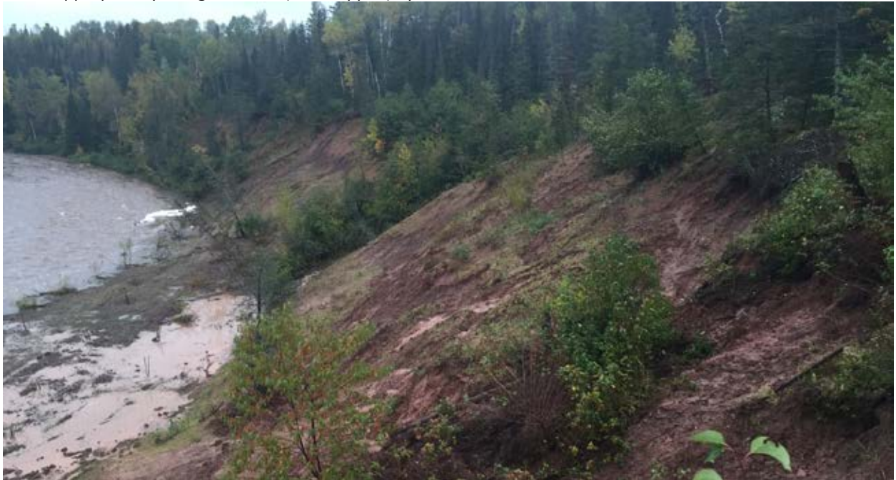
Figure 5-5 - Representative image of stabilization (bankfull bench). As illustrated in the photograph the created bankfull bench was appropriately being accessed (over-topped) by a near bankfull flow event. Date 09/24/2015.
