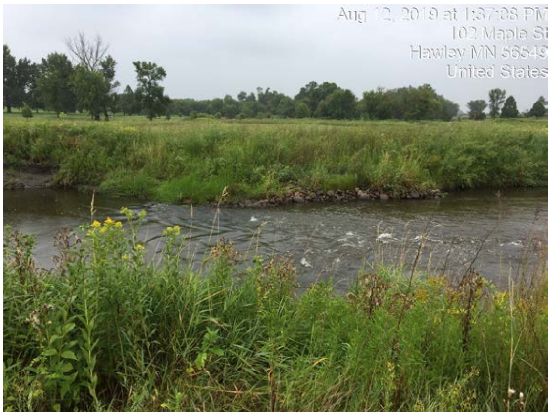
Photo 17-1. Buffalo River constructed riffle. Photo taken by Anna Varian during site visit (8/12/2019).
