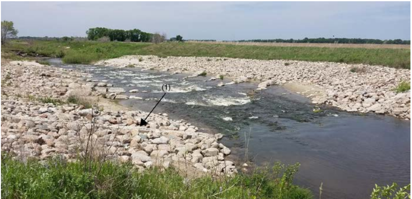
Photo 16-5 Sand Hill River fishway ramp #1 after the original drop structure was modified for fish passage. Note the cut-off weir/sheet pile in the foreground (1). Photo taken by Ed Matthiesen during site visit (6/4/2019).
