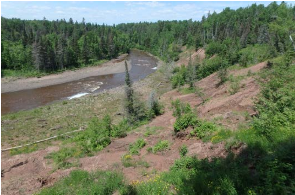
Photo 5-2 View of the project site with installed bankfull bench, July 10, 2018, two and a half years after installation.
