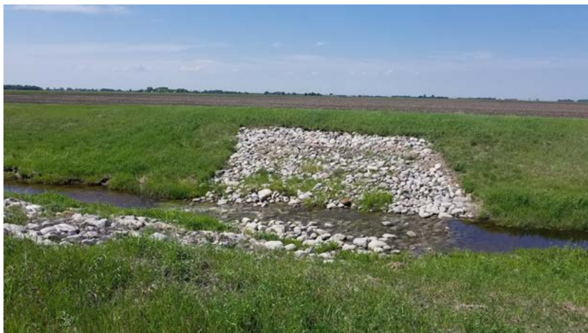
Photo 14-2 View of Burnham Creek riffle #3. Creek is 1-2 channel widths upstream (right) and 2-5 channel widths downstream (left). It is recommended to add live stakes. Photo taken by Ed Matthiesen during site visit (6/4/19).
