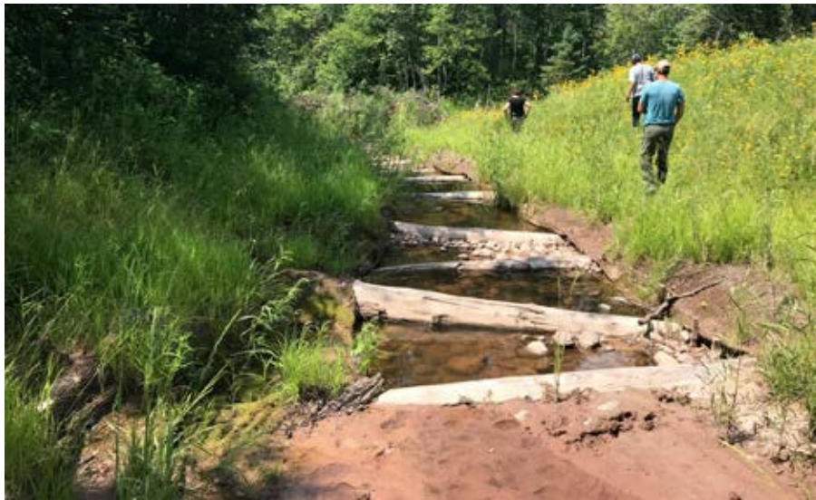
Photo 1-4 Log grade control structures near the confluence with Deer Creek. These structures are intercepting some sediment and are providing small pool habitat for aquatic organisms. Photo taken by Mike Majeski on 7/23/2019.
