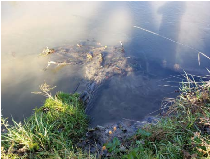
Photo 29-8. Example of the rootwads installed into the bank on the lower third of the project reach to provide some habitat complexity. Photo taken on 10/18/19 by Mark Prankus, Cardno.
