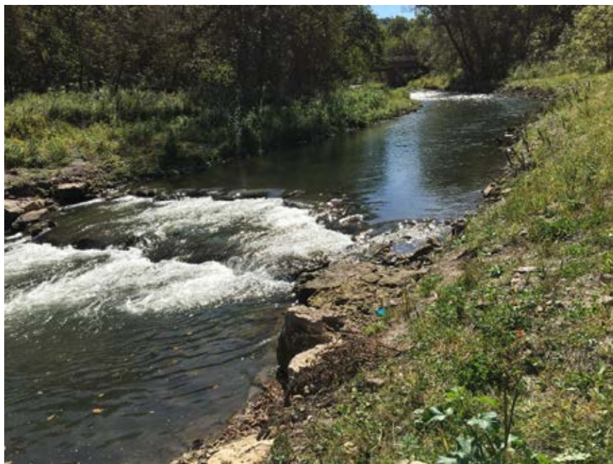
Photo 36-2 Looking upstream at reconstructed boulder vane 1. Photo taken during site visit 9/16/19 by Anna Varian
