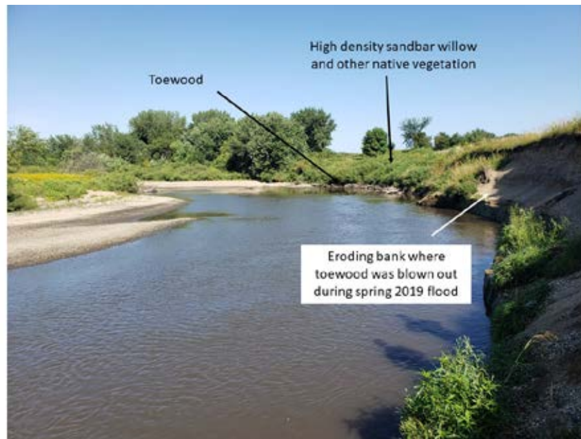
Photo 27-3. Looking upstream at the Downstream Bank (Bank 3). The upstream portion of the bank demonstrates the existing toewood used to stabilize the bank. Above the toewood, sandbar willow have colonized the lower and upper banks. At the top of the bank, primarily smooth brome and other comprise the majority of the cover. Approximately the last 150 feet of toewood blew out during spring 2019 flooding. (Photo taken 8/22/19 by Mark Prancus, Cardno).
