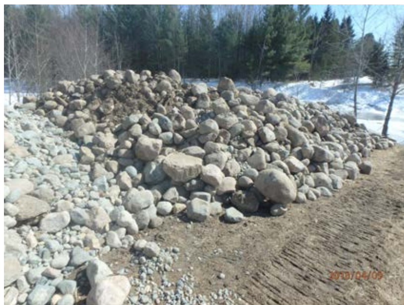
Photo 26-2. Example of the stone material installed at the County Rd 98 riffle location in 2018. Material is similar to what is naturally found in the adjacent areas of the Rat Root River. Photo provided by Koochiching County SWCD.
