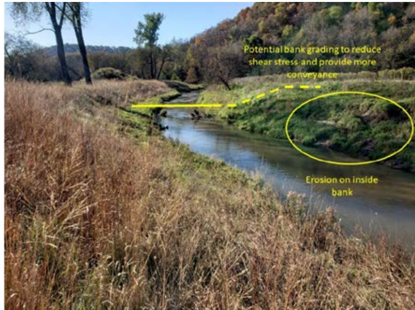
Photo 29-5 Example of looking downstream at the lower third of the project. A bench is forming on the left downstream bank where sediment is depositing on top of riprap. The dashed line represents where grading could have occurred to further improve floodplain connection and promote stream stability. Photo taken on 10/18/19 by Mark Pranckus, Cardno.
