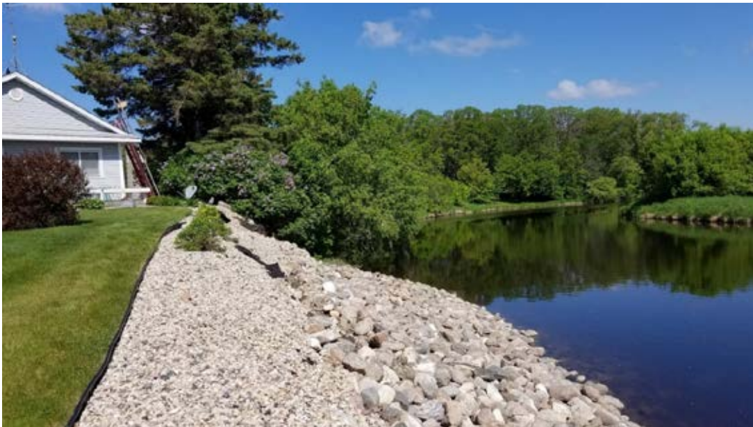
Photo 12-2 Downstream view from 0+50. There is a slope failure present on the upper slope resulting from a freeze-thaw or a quick drop in water level. It is recommended to add biological improvements. Photo taken during site visit 06/05/2019.
