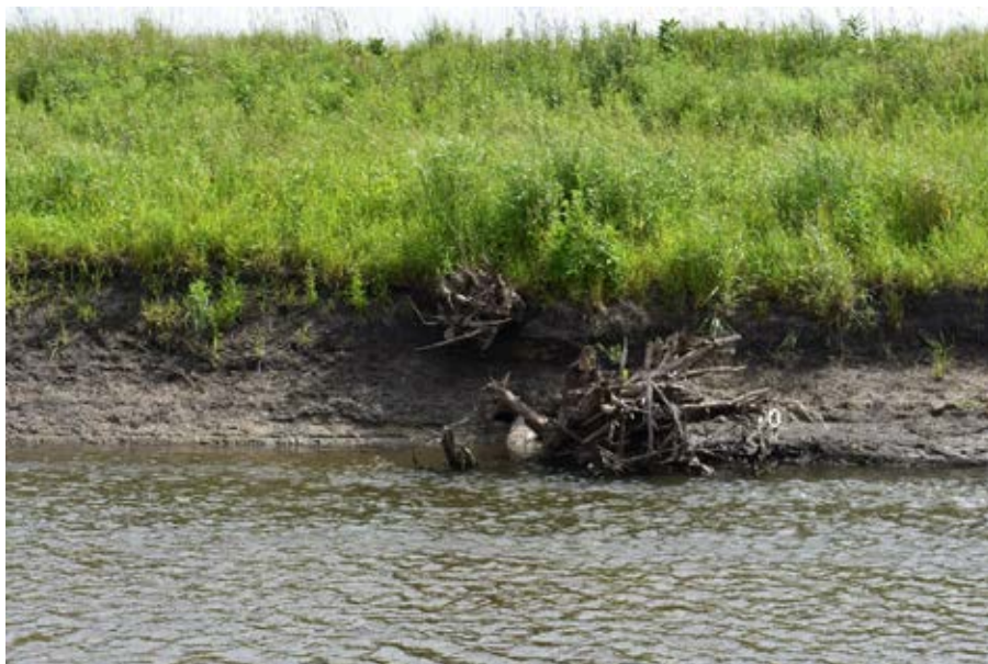
Photo 3-2 View of Elm Creek project showing a single exposed rootwad. Evaluator recommends rock/boulders on both sides of the rootwad near station 7+00 to prevent bank scour behind the rootwad. Photo taken by Ed Matthiesen during site visit (8/13/19).
