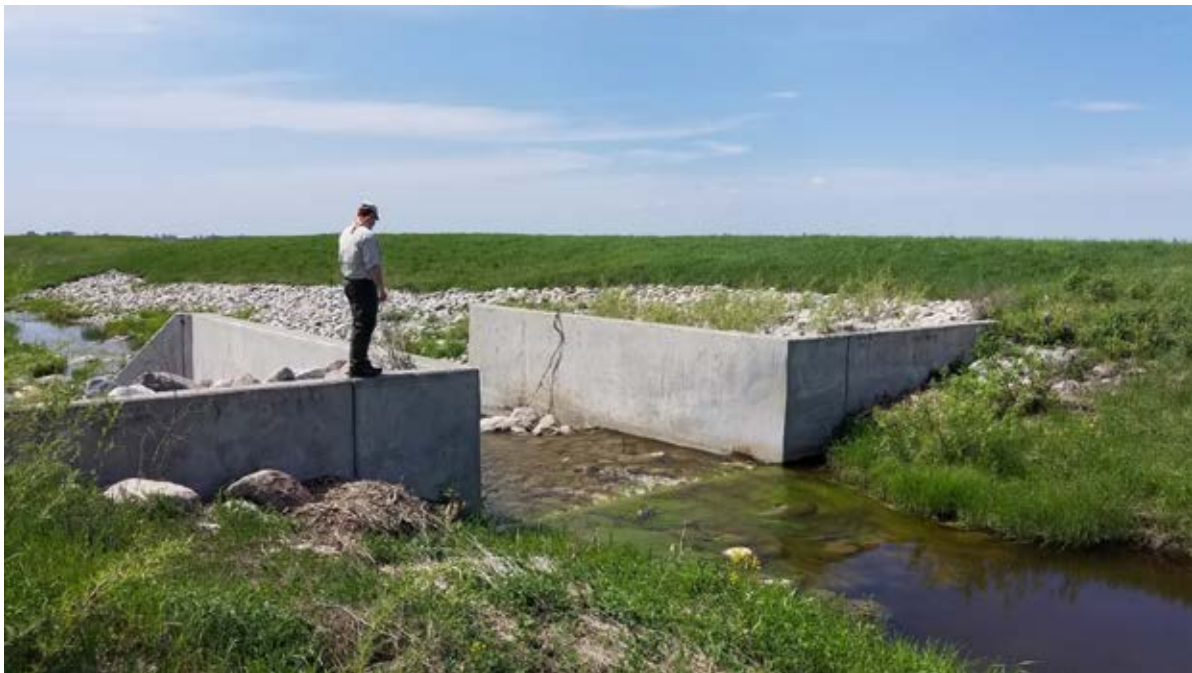
Photo 14-6 Upstream view of NRCS Rock Flume at project location 1502+00 on Burnham Creek. It is recommended to reduce the rise of the structure to less than 12 inches. Photo taken by Ed Matthiesen during site visit (6/4/19).
