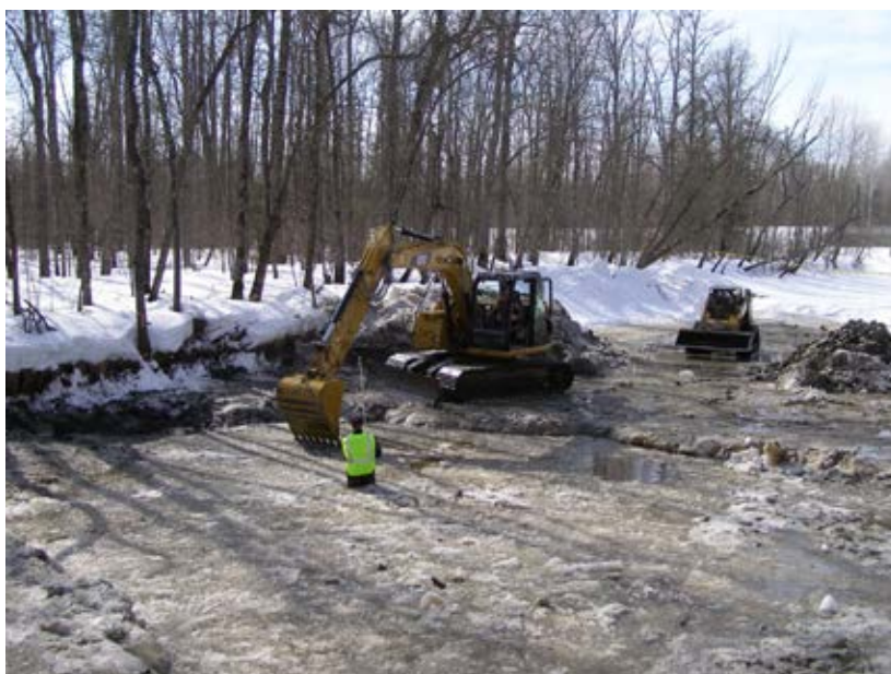
Photo 26-1. Example of riffle construction of Riffle No. 1 during winter 2013. Excavator and skid steer are operating on a frozen Rat Root River. Photo provided by Koochiching County SWCD.
