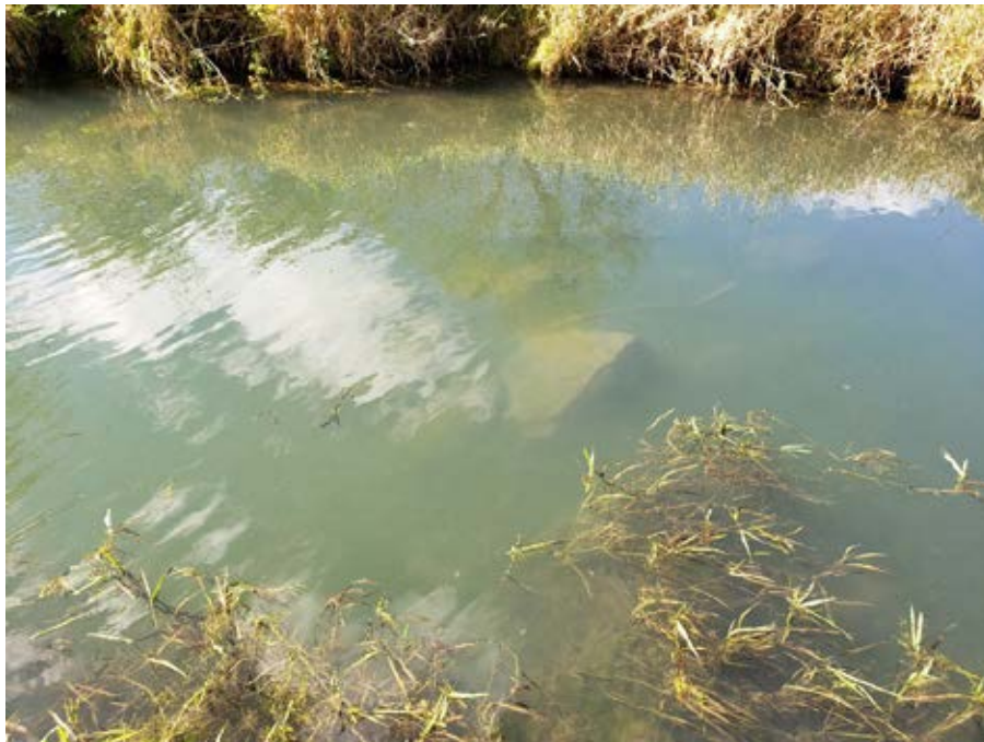
Photo 22-6. Example of a random boulder cluster used to provide in-stream cover for feeding trout. Photo taken 10/17/19 by Mark Prankus, Cardno.
