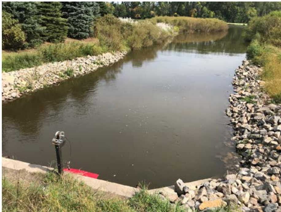
Photo 32-12 Looking downstream as Wedge Creek enters Fountain Lake. The winch and pulley with red bracket of the electric fish barrier is visible on the apron of the box culvert. (Wedge Creek – Reach 1, photo taken by Lucius Jonett during site visit 09/20/2019).
