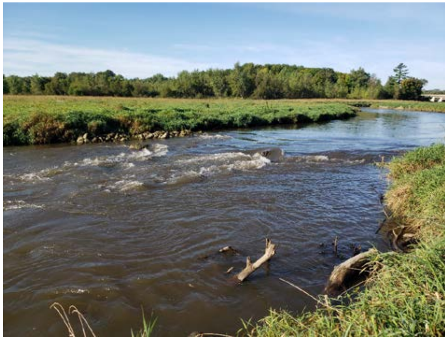
Photo 34-1 Example of a boulder J-hook near the upper third of the channel through the former Lake Shady bed. Water levels were elevated during the site assessment. Photo taken 9/16/19 by Mark Prancus, Cardno.
