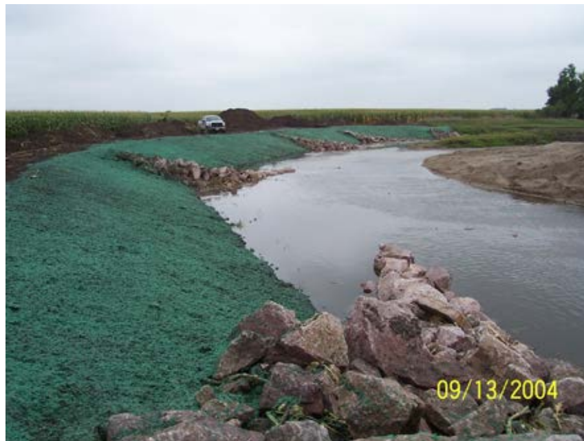
Photo 28-2. Looking upstream at the upstream project area following construction in 2014 showing five of the six rock J-hook vanes. The areas between the vanes were graded to a 3:1 slope hydroseeded with native seed mix. Notice when compared to Photo 28-1, the elevation of rock on several structures have decreased, potentially due to rock moving during high flows. Photo provided by Scott Ralston (USFWS)
