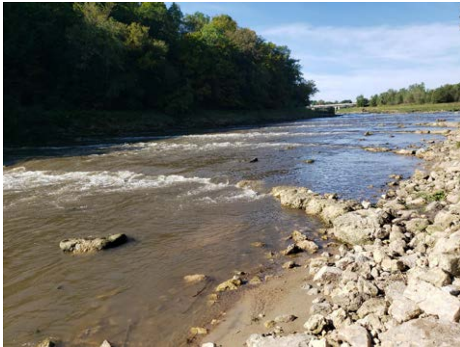
Photo 34-4 View looking upstream from streamside of the rock arch rapids. The structures are installed in an arch facing upstream and also in elongated “U” shaped in the cross section to keep turning flows into the center of the channel as water elevation increases, which reduces bank erosion potential. Photo taken 9/16/19 by Mark Pranckus, Cardno.
