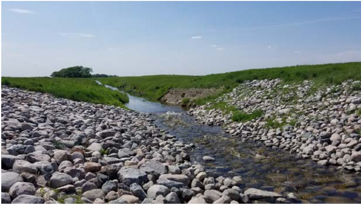
Photo 14-3 View of Burnham Creek riffle #4. Creek is 1-2 channel widths upstream (right) and 2-5 channel widths downstream (left). It is recommended to add live stakes to 2 channel widths downstream. Photo taken by Ed Matthiesen during site visit (6/4/19).
