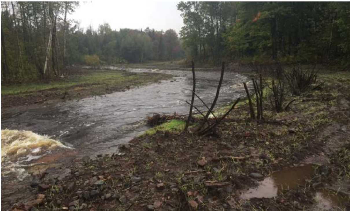
Photo 9-9 Representative image of project elements: Toe Wood (right) with willow harvested mats above and Log J Hook with Rootwad downstream (left) 09/24/2015.
