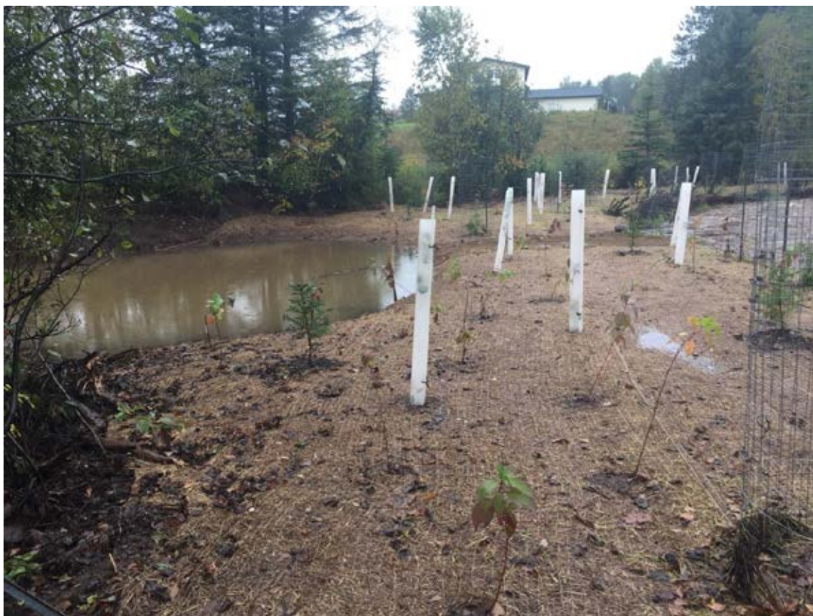
Photo 10-5 A constructed offline "wildlife pond" (left side of image), a minor project change, was a product of balancing cut & fill. Date 10/24/2015.
