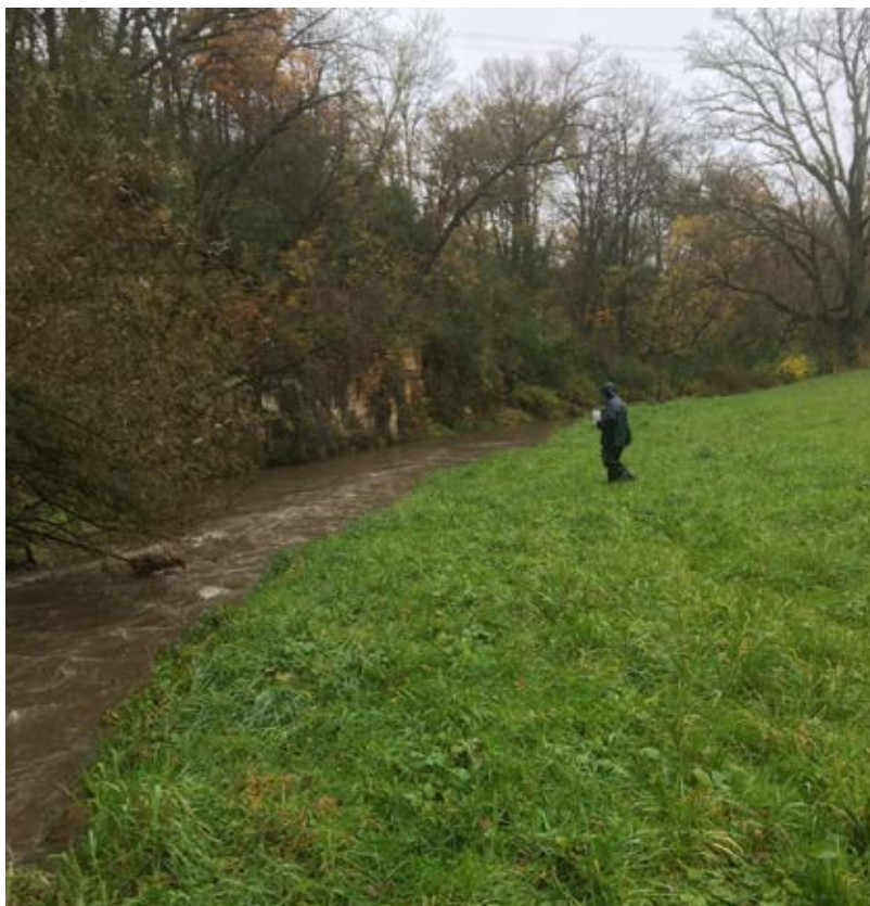
Photo 35-3 Middle Branch Whitewater River, area where stream width was reduced, banks were re-shaped and rock added to banks. Photo taken 10/21/2019 by Anna Varian.
