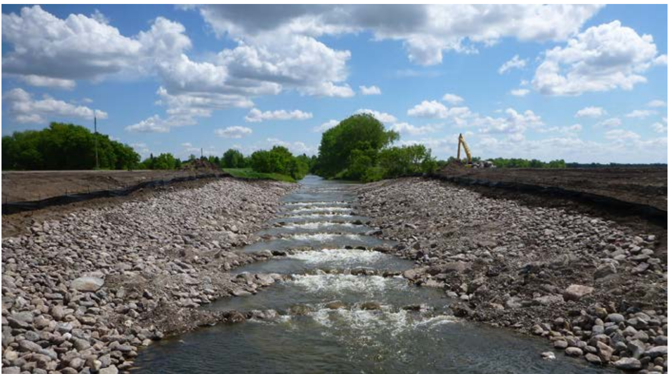
Photo 16-4 Photo of drop structure 4 after construction of fishway. Photo provided by project partners (taken 5/26/2017)
