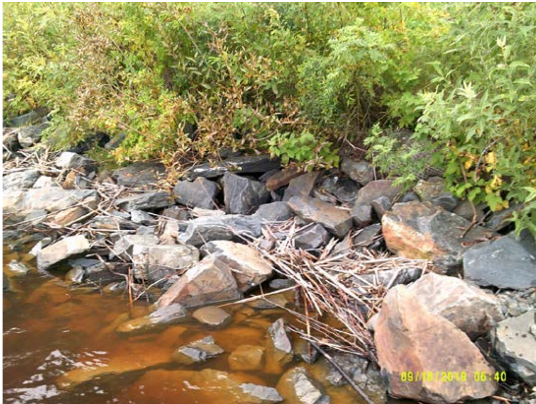
Photo 25-7. Example of rock toe and vegetated bank at the Fish Camp Site. Photo taken during site visit 9/18/2019.
