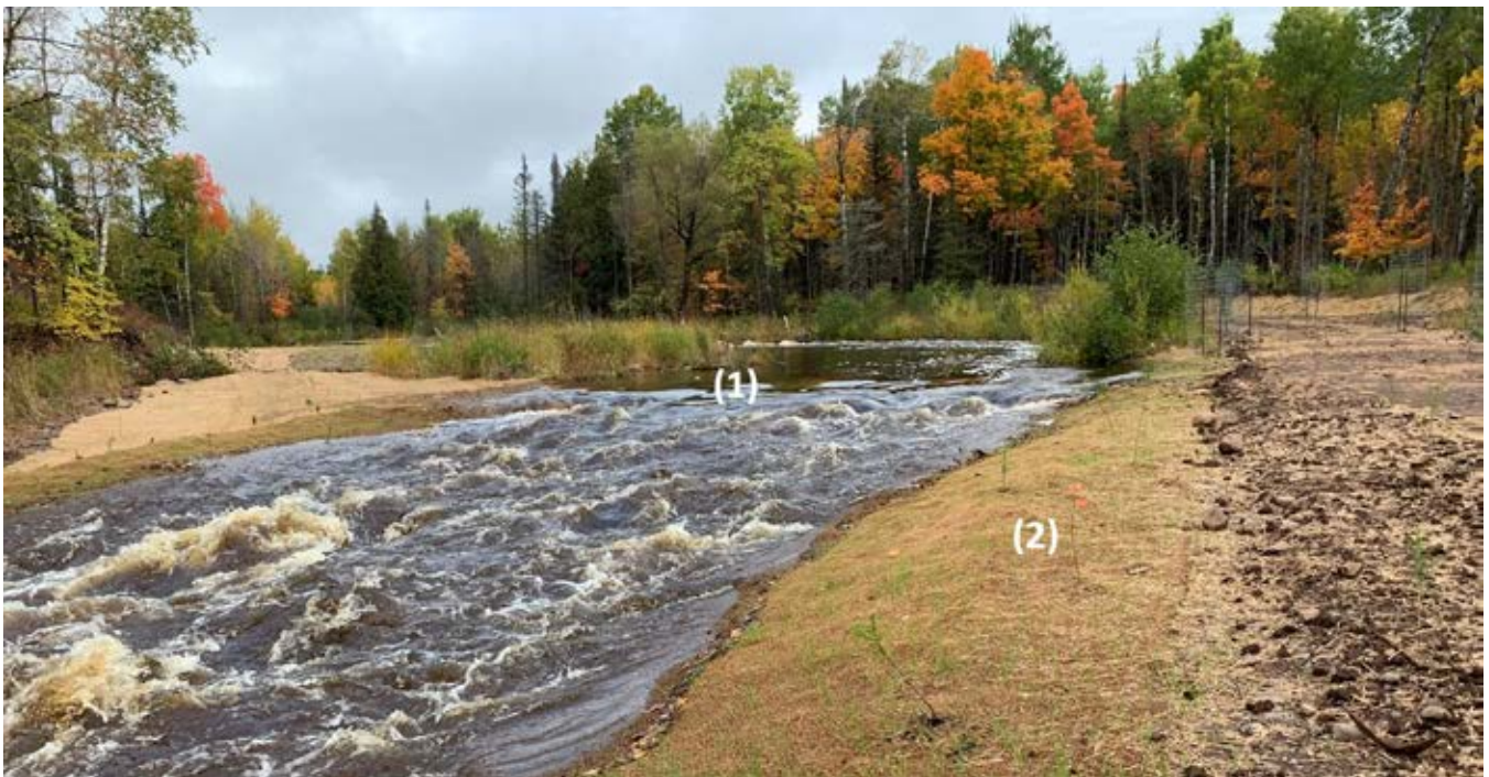
Photo 9-6 Representative image of high gradient segment of river and repaired grade control structure (1) looking upstream. Note saplings recently planted along stream edge (2). Photograph taken by Kevin Biehn during 10/1/2019 site visit.
