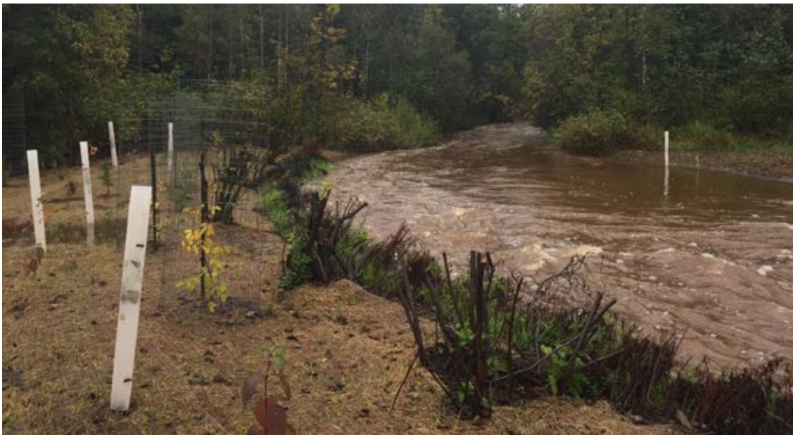
Photo 10-4 Representative image of toe wood (near bank) and onsite transplants (near bank) along with the tree and shrub plantings with browse protection. Date 10/24/2015.
