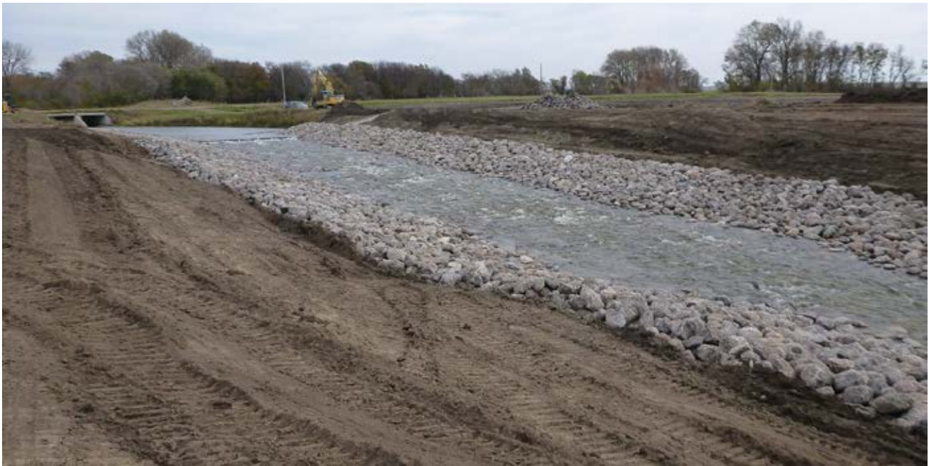
Photo 16-3 Drop structure 4 during construction of fishway. Photo provided by project partners (taken 10/14/2019).
