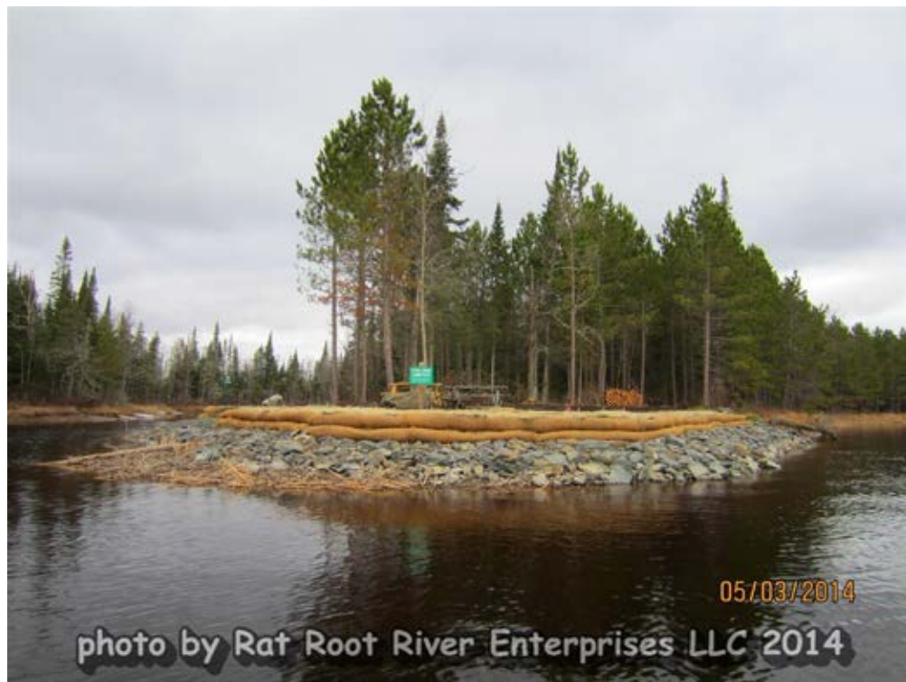
Photo 25-2. Example of the Fish Camp bank stabilization site in spring 2014 following construction in fall 2013. Photo provided by Ed Lombard, Rat Root River Enterprises, LLC.
