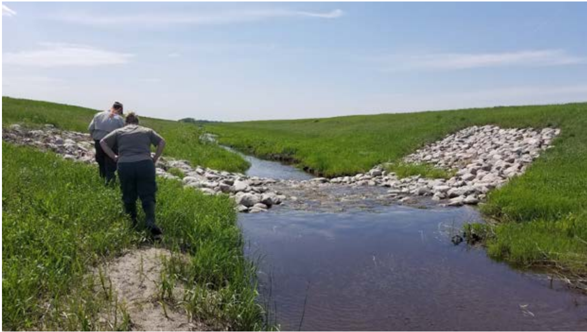
Photo 14-5 Upstream view of riffle #8. Creek is 1-2 channel widths upstream (front) and 2-5 channel widths downstream (back). This riffle is meeting project goals of reducing bank erosion. Photo taken by Ed Matthiesen during site visit (6/4/19).
