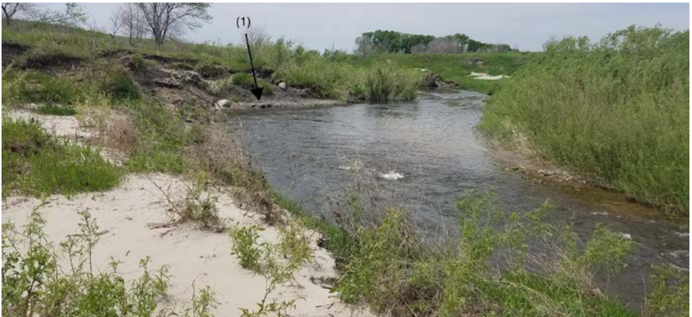
Photo 16-6 View downstream of Sand Hill River fishway ramp #1. Note the area of un-vegetated sluffing bank outside of the project area where additions of sandbar willow at the bend could increase stability (1). Photo taken by Ed Matthiesen during site visit (6/4/2019).
