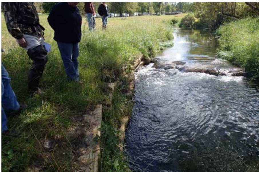
Photo 33-5 Reggraded slope, Rock deflector and Rock weir. Site visit 09/18/2012.
