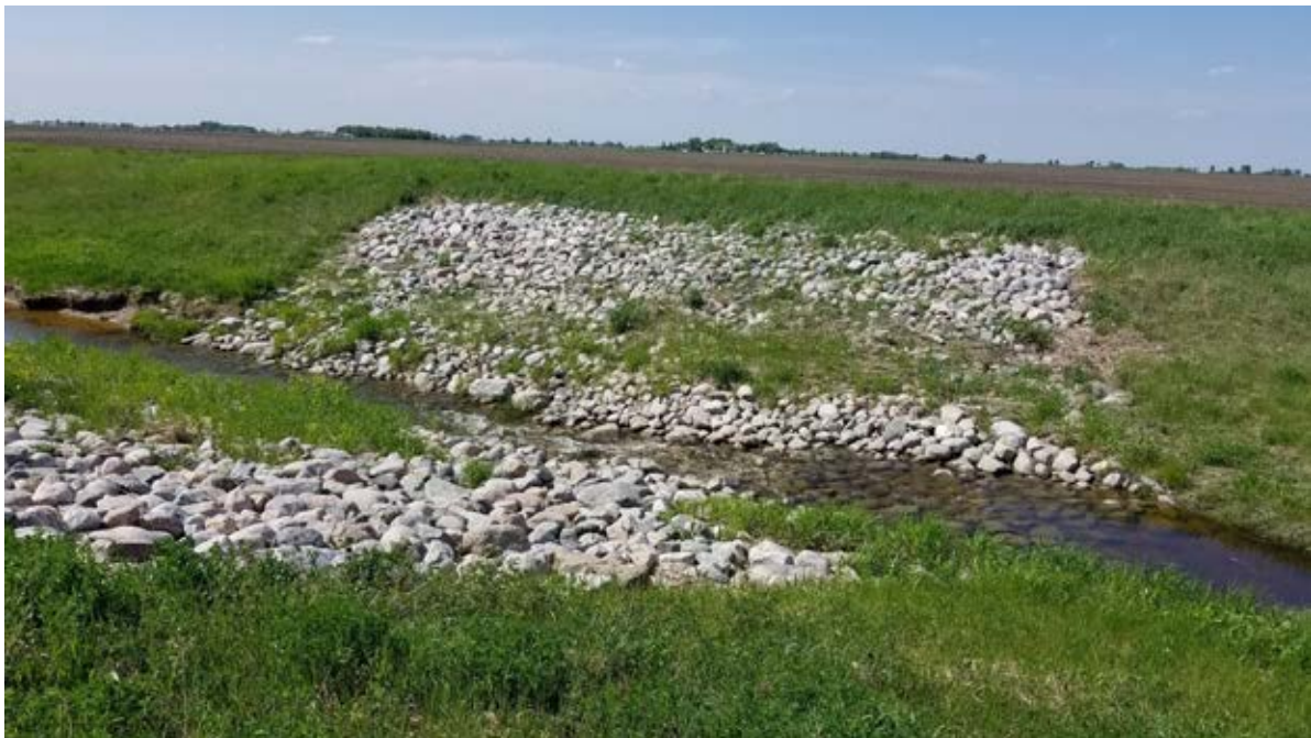
Photo 14-4 Upstream view of riffle #5. Creek is 1-2 channel widths upstream (right) and 2-5 channel widths downstream (left). It is recommended to add live stakes. Photo taken by Ed Matthiesen during site visit (6/4/19).
