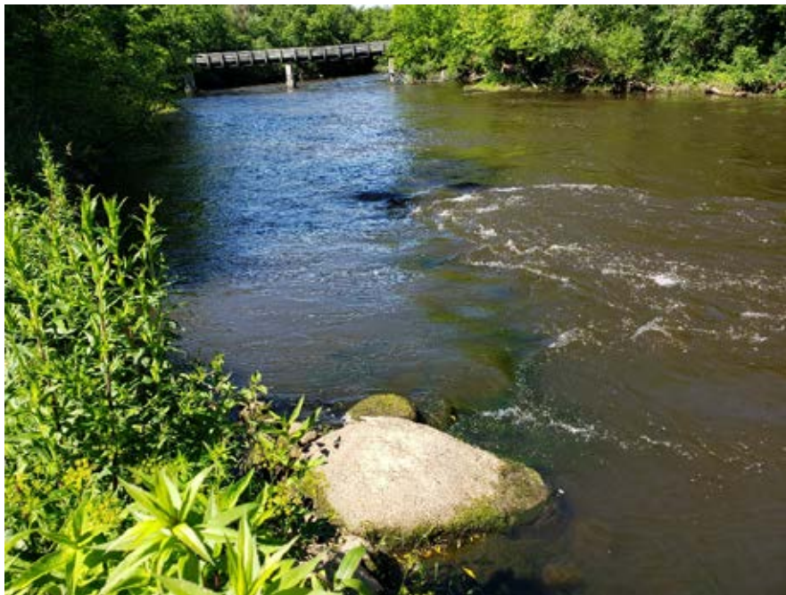
Photo 30-6 – Looking upstream at the upstream stream barb from the toewood bench. The majority of the stones for the barb are submerged, but are deflecting flow to the center of the channel and away from the treatment bank. (Photo taken 6/26/19 by Mark Prankus, Cardno).
