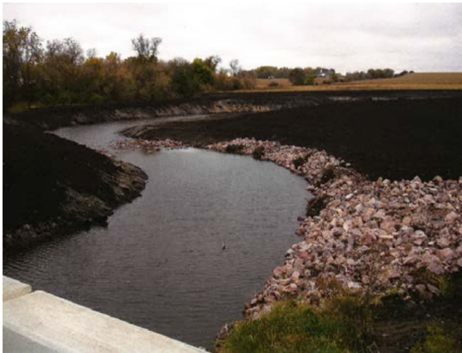
Photo 3-1 View of Elm Creek project from County Highway 36 bridge after construction and before vegetation establishment. Site evaluator questions the intended effect of rootwad placement in riprap and the elevation that the rootwads were installed. Photo taken during construction (2014).
