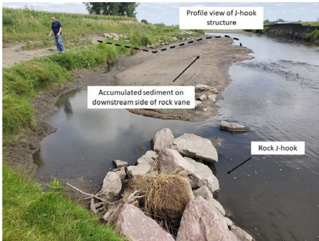
Photo 28-5. Looking upstream at the downstream project area. The two rock J-hook vanes installed in the project area can be seen. A large amount of sediment has accumulated between the structures, which helps to build the bank and protect against erosion. If the upstream vane angle was greater and extended into the channel more, the sediment in the hook of the vane would likely be scoured out, creating pool habitat. (Photo taken 8/22/19 by Mark Prankus, Cardno).
