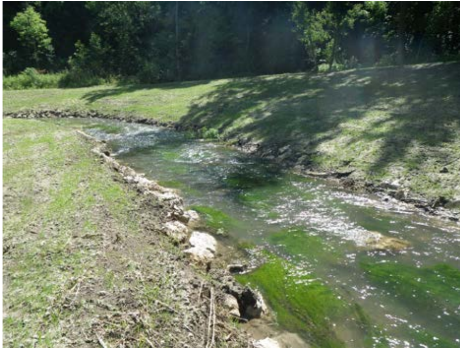
Photo 22-9. Example of Pickwick Creek following construction in 2011. Banks were seeded and straw mulched. The low bank on the left helps to reduce shear stress on the outside bend during high flows. Photo taken August 2011 and provided by MN DNR.
