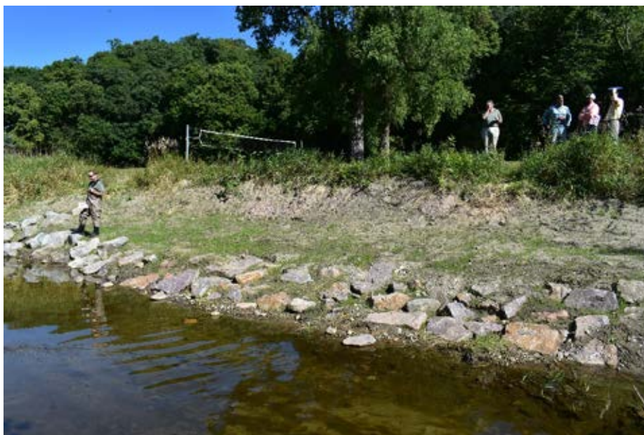
Photo 31-10 Bank regrading creating floodplain terrace within the incised channel completed during final streambank maintenance activities in August 2019. (Seven Mile Creek County Park, photo taken during site visit 08/30/2019).
