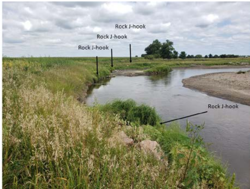
Photo 28-1. Looking upstream at the upstream project area. Locations of four of the six rock J-hook vanes are identified. Vegetation along the bank is 3 to 4 feet tall and well-established. (Photo taken 8/22/19 by Mark Prankus, Cardno).
