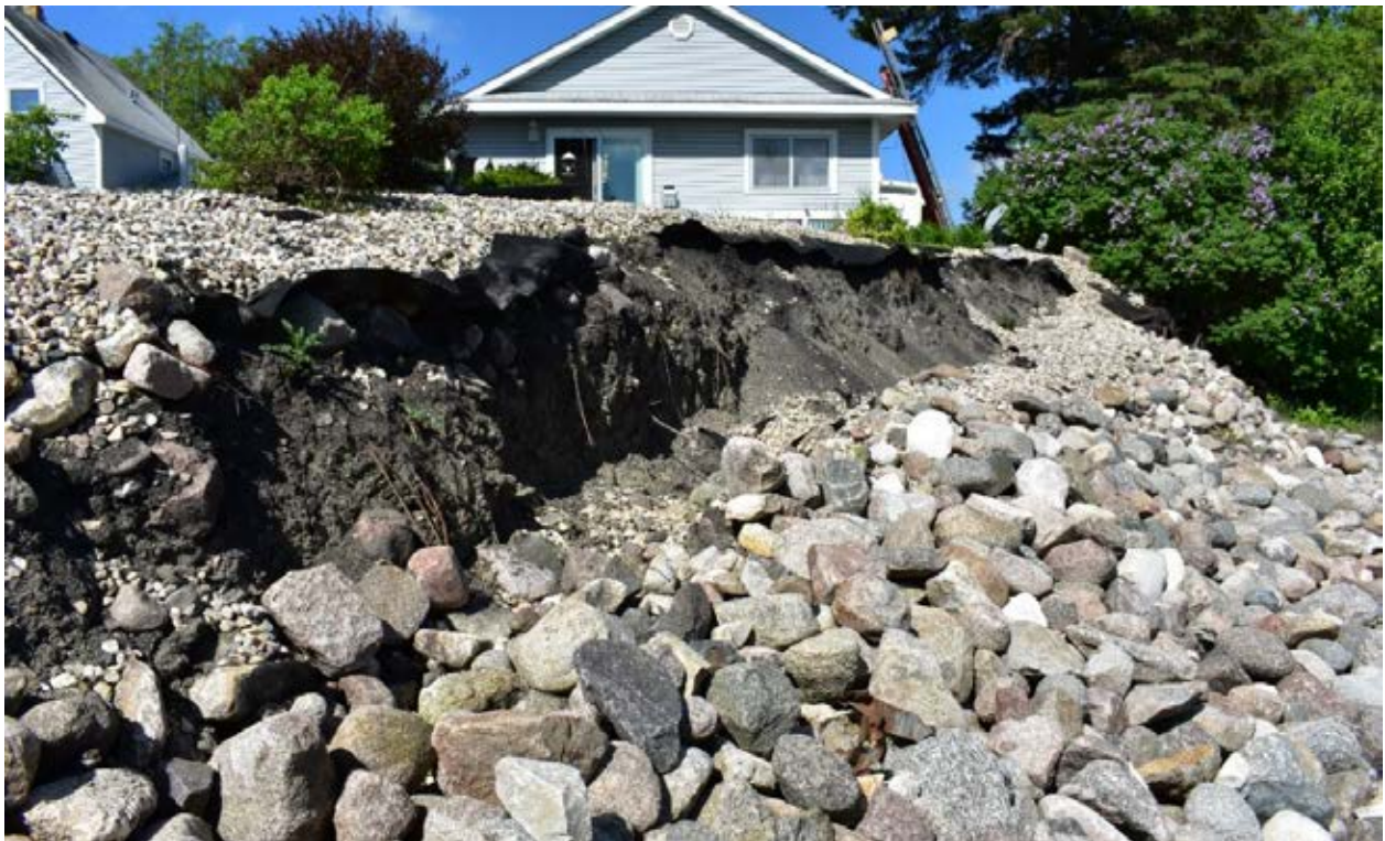
Photo 12-4 View of the disturbance at the top of the streambank which may be signs of a rotational failure or slump. Regrading of this ridge back toward the homes is recommended along with revegetation on the new slope. Photo taken during site visit 06/05/2019.
