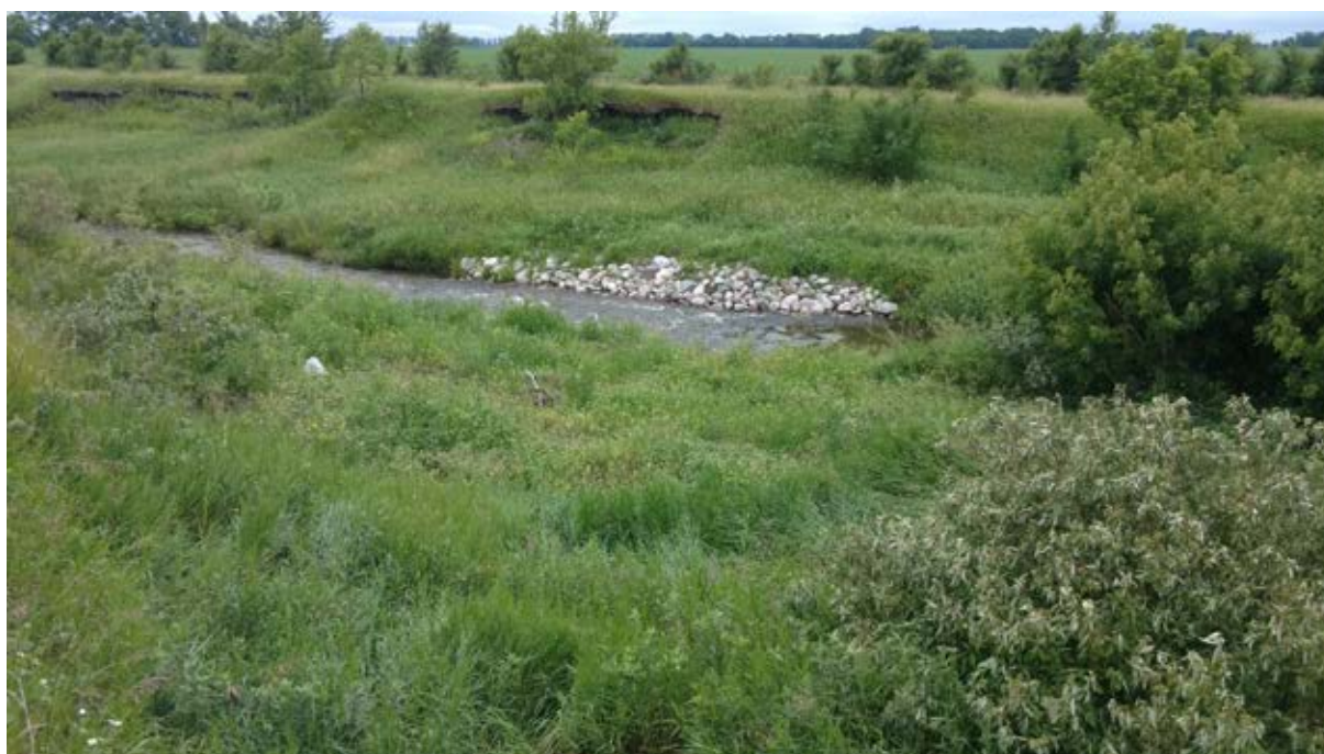
Photo 15-2 View of constructed riffle at project station 91+85. Pre-existing bank slump failures are still visible in the background. Photo taken by others during a post-construction, final inspection (6-29-2017).
