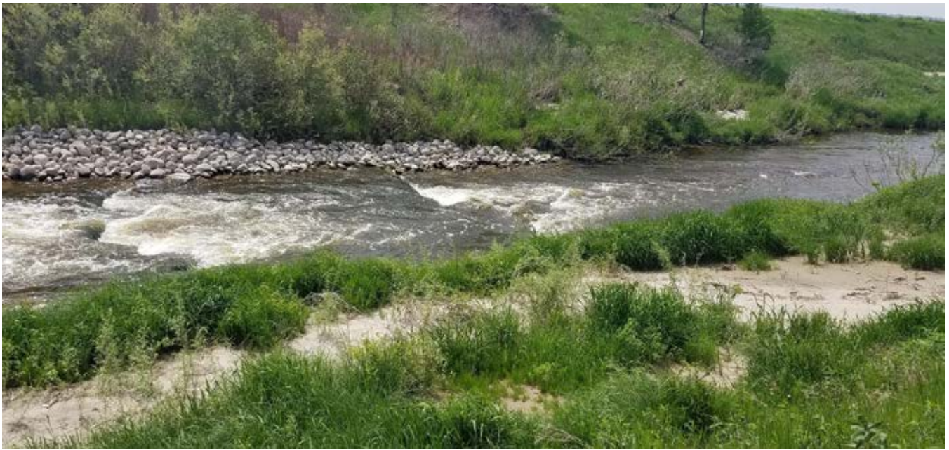
Photo 16-9 Sand Hill River fishway ramp #3 after the original drop structure was modified for fish passage. Shrubs at downstream end are holding the soil in place. Photo taken by Ed Matthiesen during site visit (6/4/2019).
