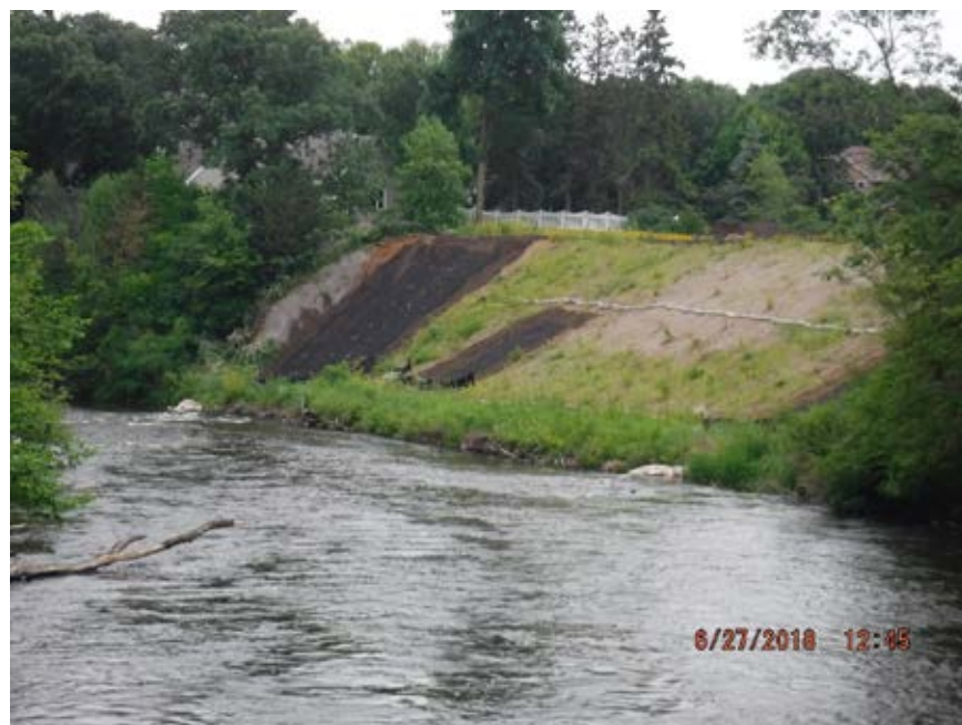
Photo 30-2. View looking downstream to the project area on the right hand side of the image after follow-up planting where vegetation had not established and robustly. (Photo provided by project partners, taken 6/27/2018).
