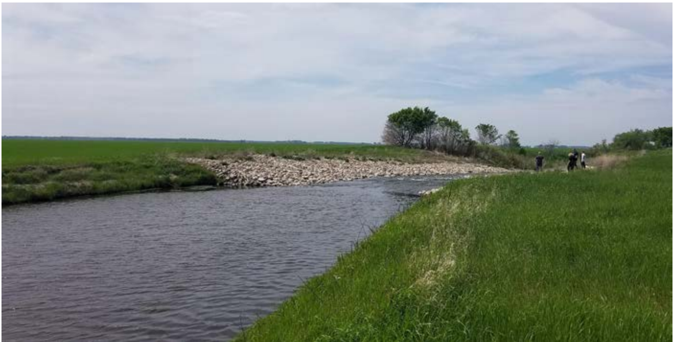
Photo 16-10 Upstream view of fishway ramp #3 with well-established vegetation and no noted erosion on the banks. Photo taken by Ed Matthiesen during site visit (6/4/2019).
