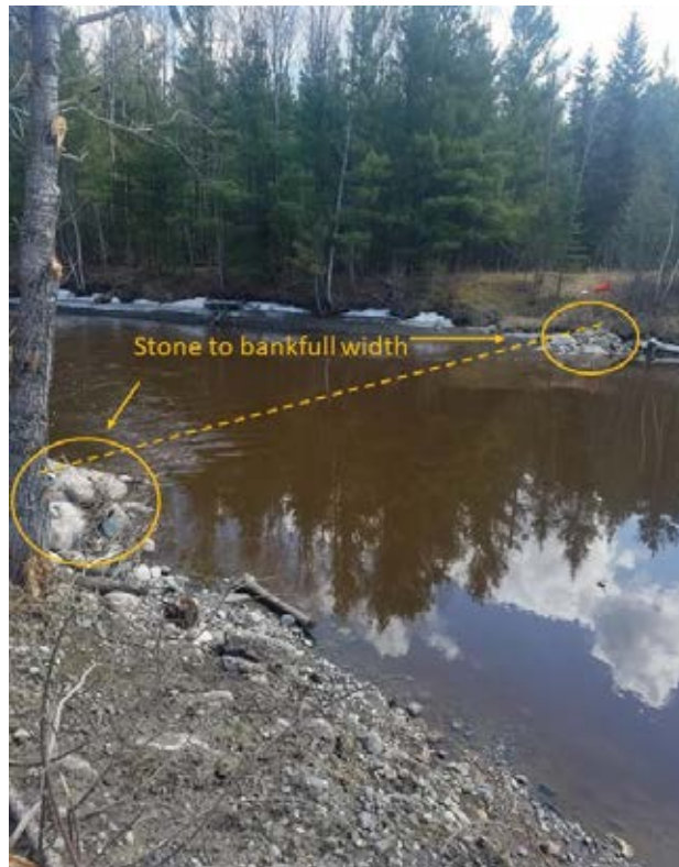
Photo 26-4. Example of a completed constructed riffle. The stone extends to the bankfull width and is throughout the entire channel. Photo provided by Koochiching County SWCD.
