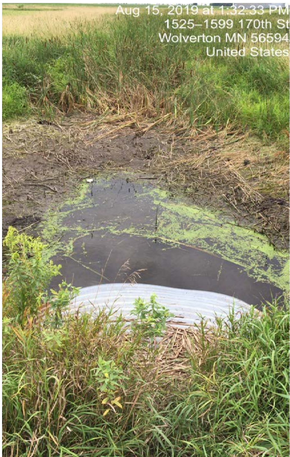
Photo 13-6. View of existing condition at a location just upstream from the Phase 1 construction. Water is stagnant and channel is choked with sediment and vegetation. Photo taken by Anna Varian during site visit (8/15/2019).
