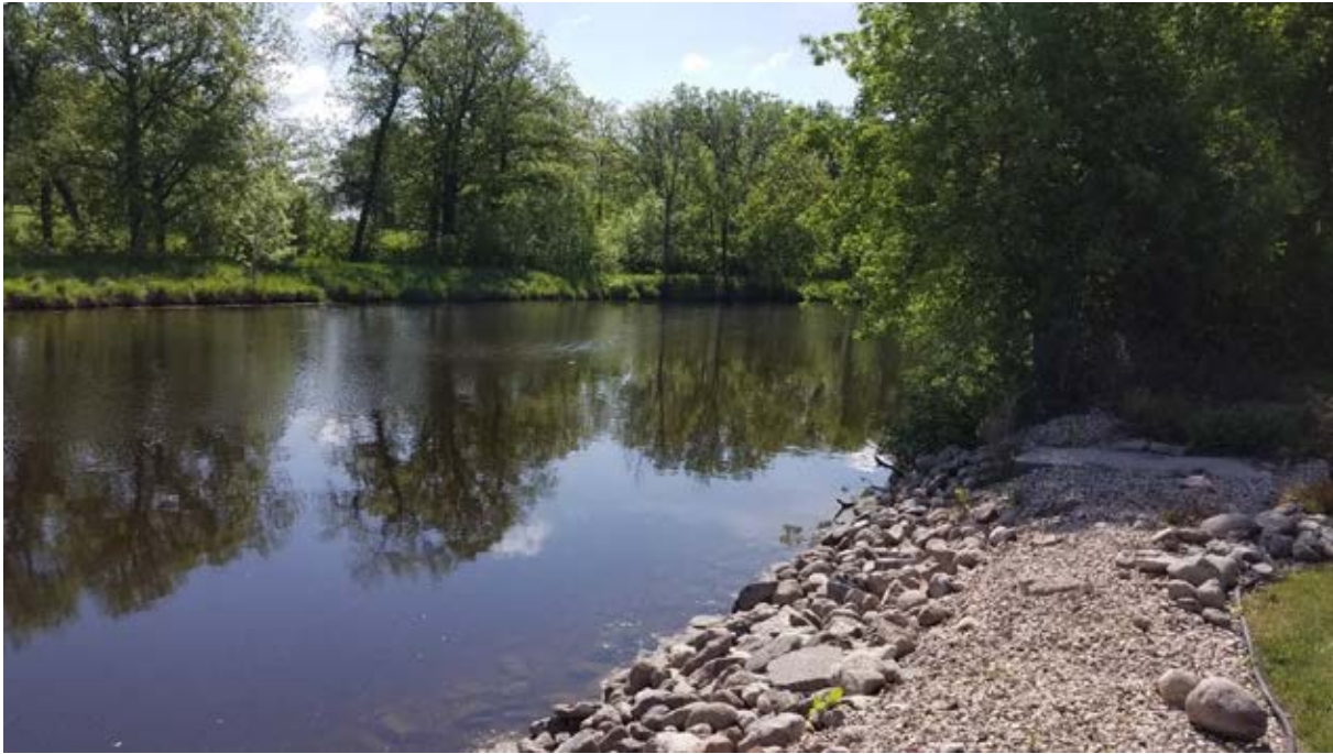
Photo 12-1 Upstream view of 0+25. It is recommended to consider vegetated riprap on slopes. Photo taken by Ed Matthiesen during site visit (6/5/2019).
