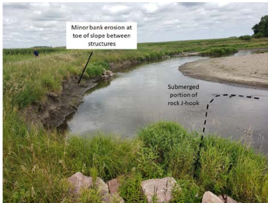
Photo 28-3. Looking upstream at the upstream project area. Minor bank erosion is occurring along the toe between J-hook vanes No. 4 and 5. (Photo taken 8/22/19 by Mark Prankus, Cardno).
