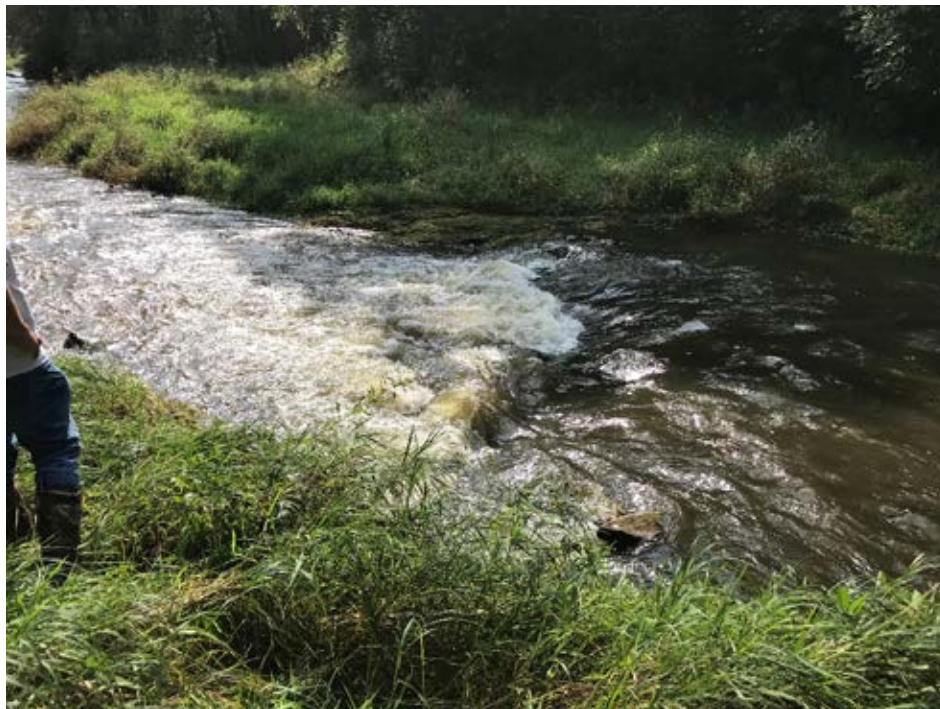
Photo 32-6 Cross log installed on the Reach 5 project of Wedge Creek. Cross log was located based on landowner input to create and maintain a wet crossing upstream of the cross log. (Wedge Creek – Reach 5, photo taken by Lucius Jonett during site visit 09/20/2019).
