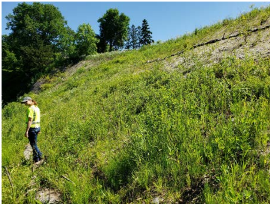
Photo 30-8. Example of vegetation development on the treatment bank. Vegetation on the bench and the lower portion of the slope are developing nicely. Bare areas on the upper slope where additional repairs were completed can be observed, but will fill in over time. (Photo taken 6/26/19 by Mark Prankus, Cardno).
