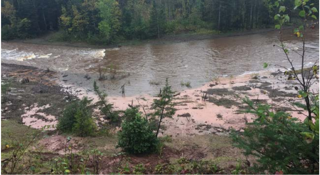
Figure 5-5 - Representative image of stabilization (bankfull bench). As illustrated in the photograph the created bankfull bench was appropriately being accessed (over-topped) by a near bankfull flow event. Date 09/24/2015.
