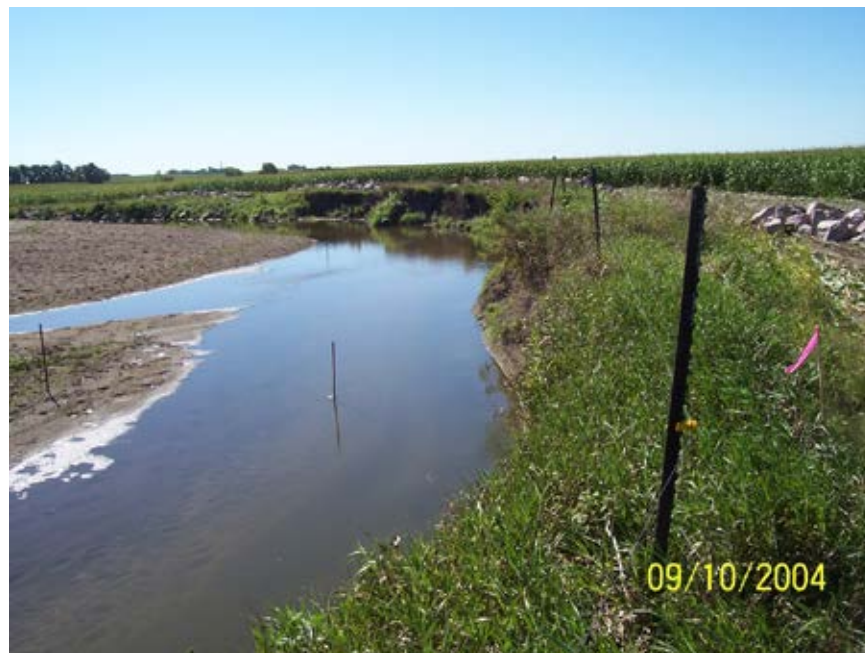
Photo 28-4. Looking downstream near the upstream end of the upstream project area prior to construction in 2014. Note the nearly vertical, severely eroding banks. Rocks used to create the J-hook vanes can be observed along the top of the bank. Photo provided by Scott Ralston (USFWS).
