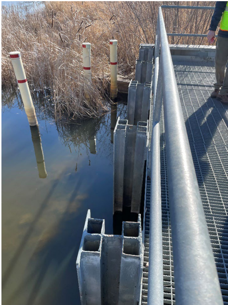
Photo 47. Typo Lake outlet barrier with barrier grates not currently in place, photo taken during site visit 3/1/24.
