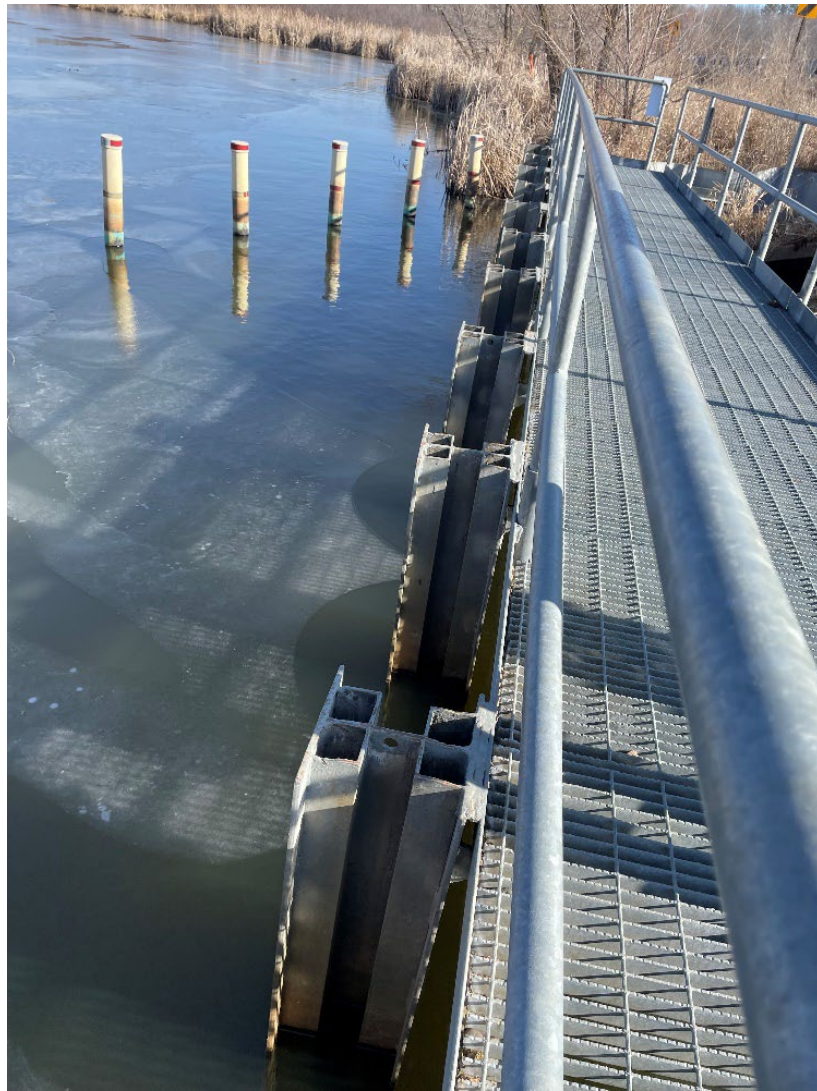
Photo 46. Typo Creek barrier with barrier grates not currently in place, photo taken during site visit 3/1/24.
