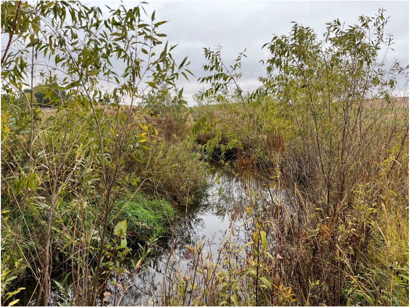
Figure 22 Restored section of Dutch Creek. Live staked willow and other wetland vegetation was well-established in the Vegetated Reinforced Soil Slope (VRSS) and installed toe wood was well-covered below water level. Site visit 10/19/2024.
