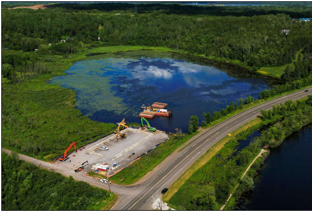
Photo 36. Example of sediment removal operations to restore Perch Lake bathymetry. Photo provided by Jeremy Pinkerton, MNDNR.
