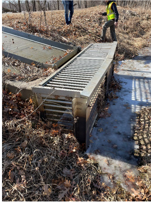
Photo 42. Barrier with retrofit at inlet of Bone Lake, photo taken during site visit 3/1/24.
