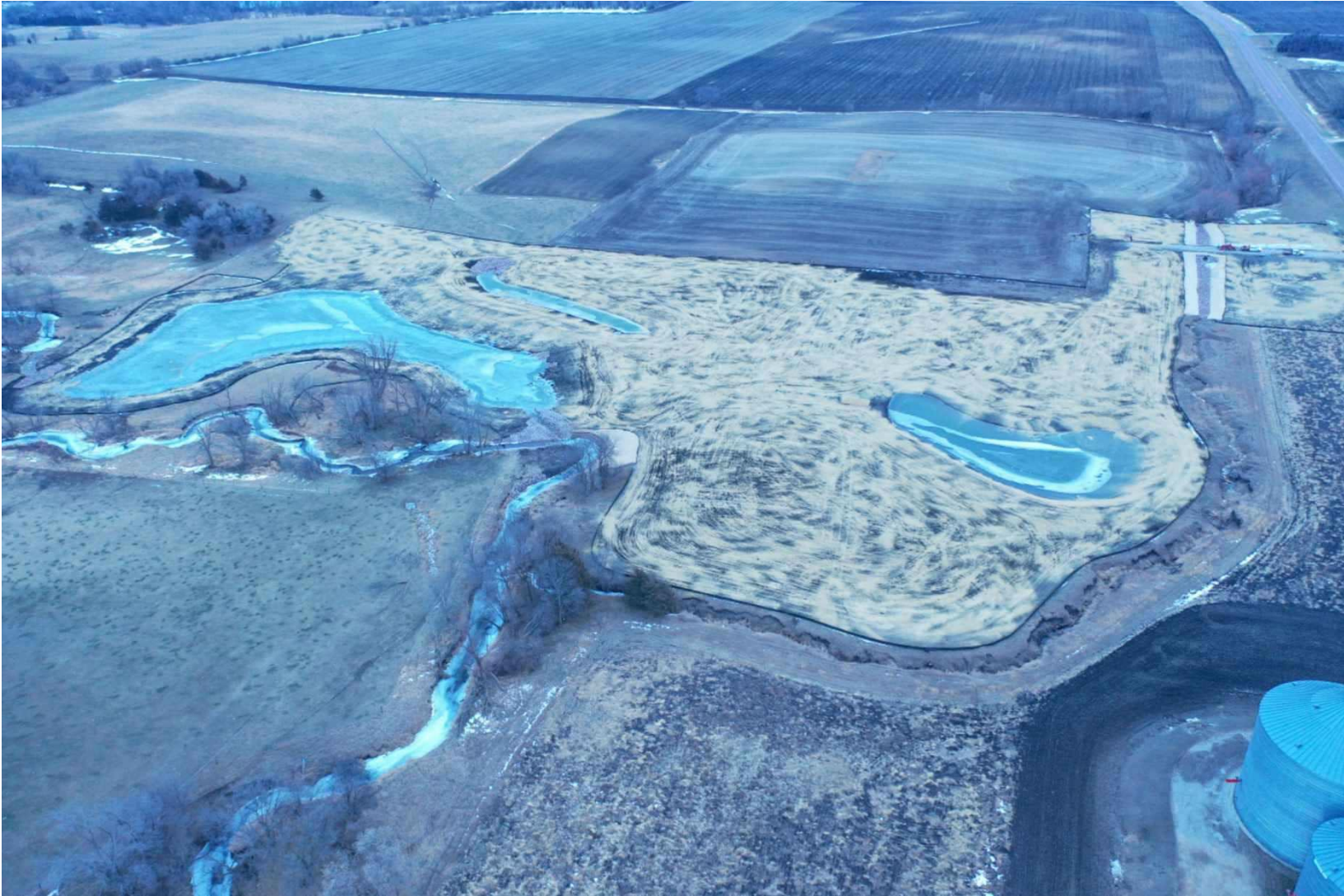
Figure 20 Aerial view of project's south lot facing south with Dutch Creek and the offline habitat wetland pond left of the image. Photo taken in December 2021.
