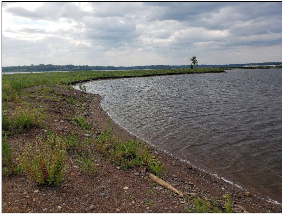
Photo 9. Example of the shoreline of the larger Grassy Point island that is within the sheltered bay. No stone toe was initially used to prevent wind and wave erosion. Photo taken by M. Pranckus (EOR) on August 17, 2023.
