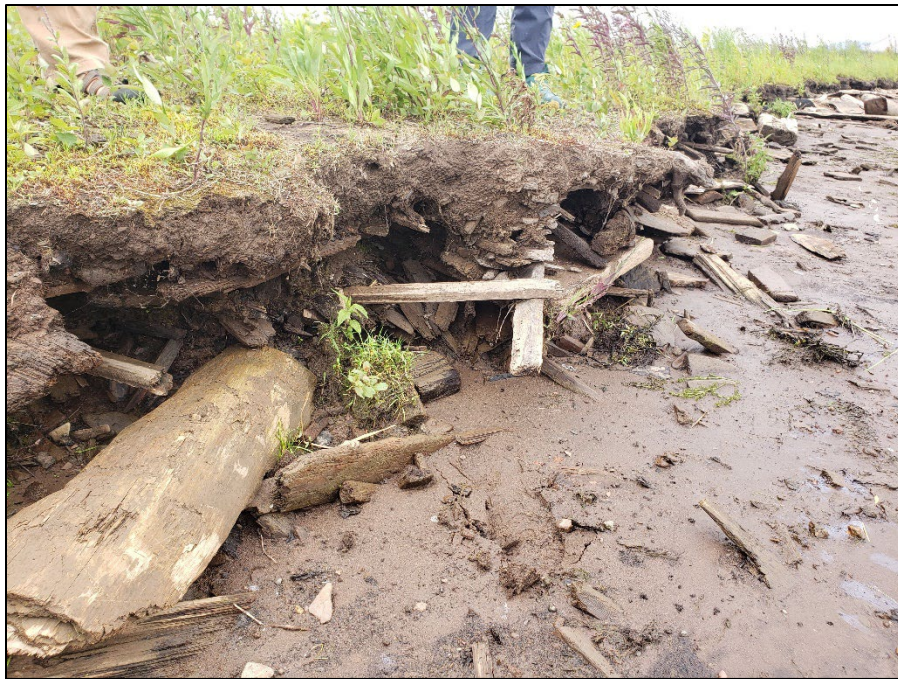
Photo 11. Example of where minor shoreline erosion is occurring on the larger Grassy Point island showing how the island was created using wood waste excavated from the project area and the top layer of biomedium excavated from Kingsbury Bay. Photo taken by M. Pranckus (EOR) on August 17, 2023.
