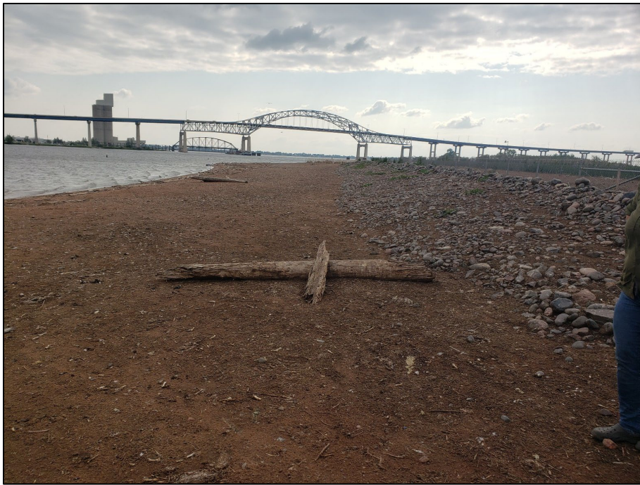
Photo 20. Looking at the shoreline of a restored Interstate Island. Driftwood and a rock berm are structures used to reduce wind and wave erosion and provide habitat for shorebirds. Photo provided by M. Pranckus (EOR) 8/17/2023.
