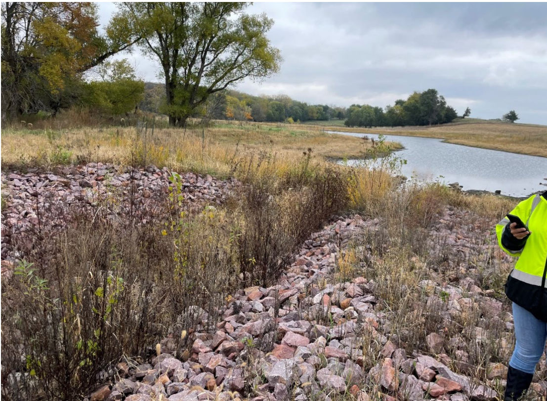
Figure 23 Rock inlet to spawning habitat wetland.
