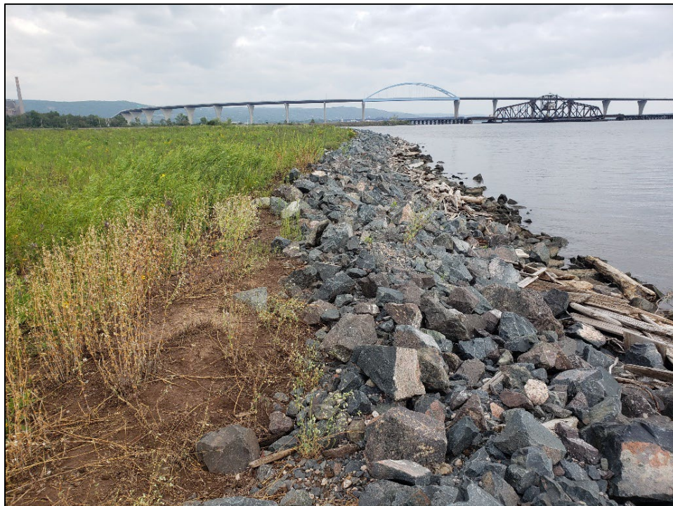
Photo 8. Example of the shoreline on the larger Grassy Point island that faces the main St. Louis River channel. A stone toe was added during construction to prevent wind and wave erosion. Photo taken by M. Pranckus (EOR) on August 17, 2023.
