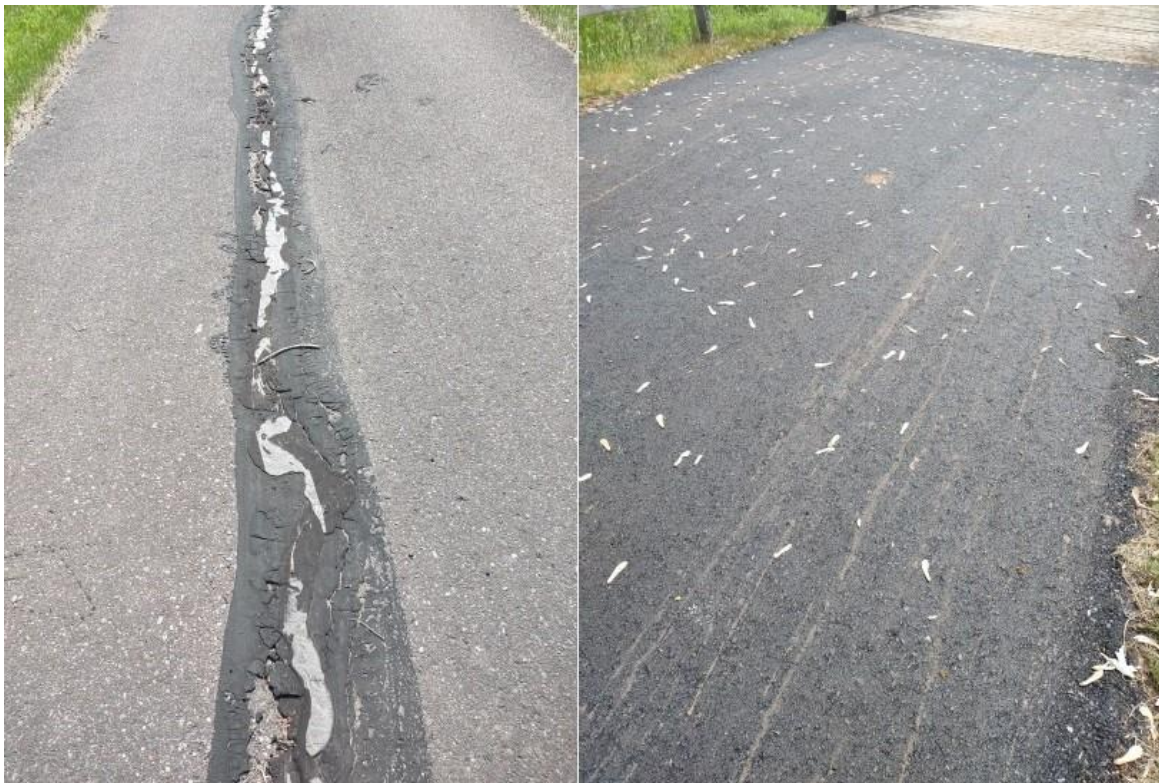
Figure 10. Cracked segment of Munger State Trail (left) that received crack sealing (right).
