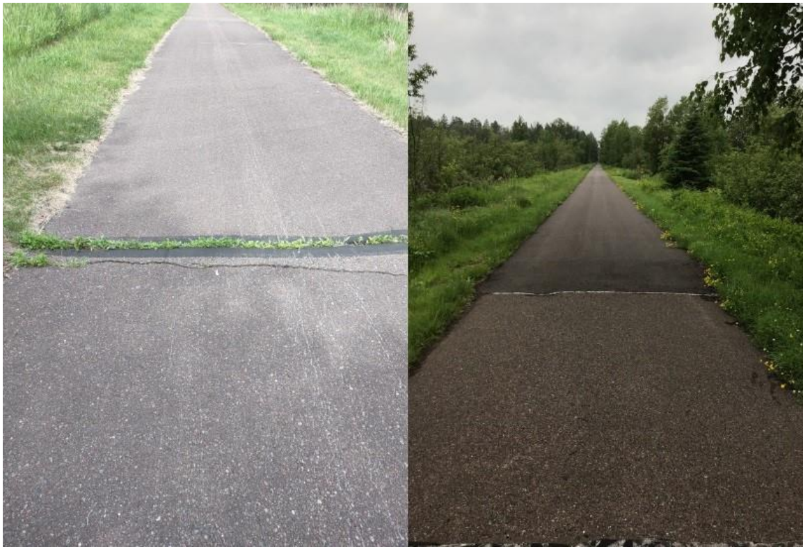
Figure 9. Cracked segment of Munger State Trail (left) that received new asphalt (right).
