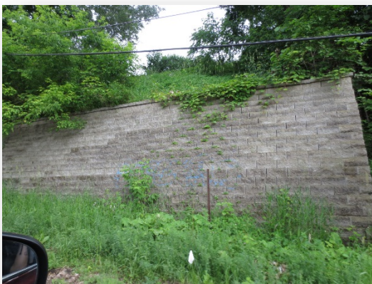
Retaining wall in St. Paul. Photo courtesy of MNDNR
