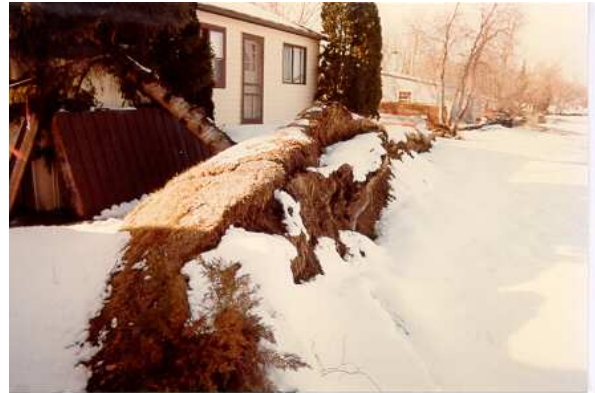
The west shore of Big Cormorant Lake, Becker County, suffered from “ice power”. Taken on March 5, 1987, this photo demonstrates that aesthetics is not the only reason structures need proper setback.
