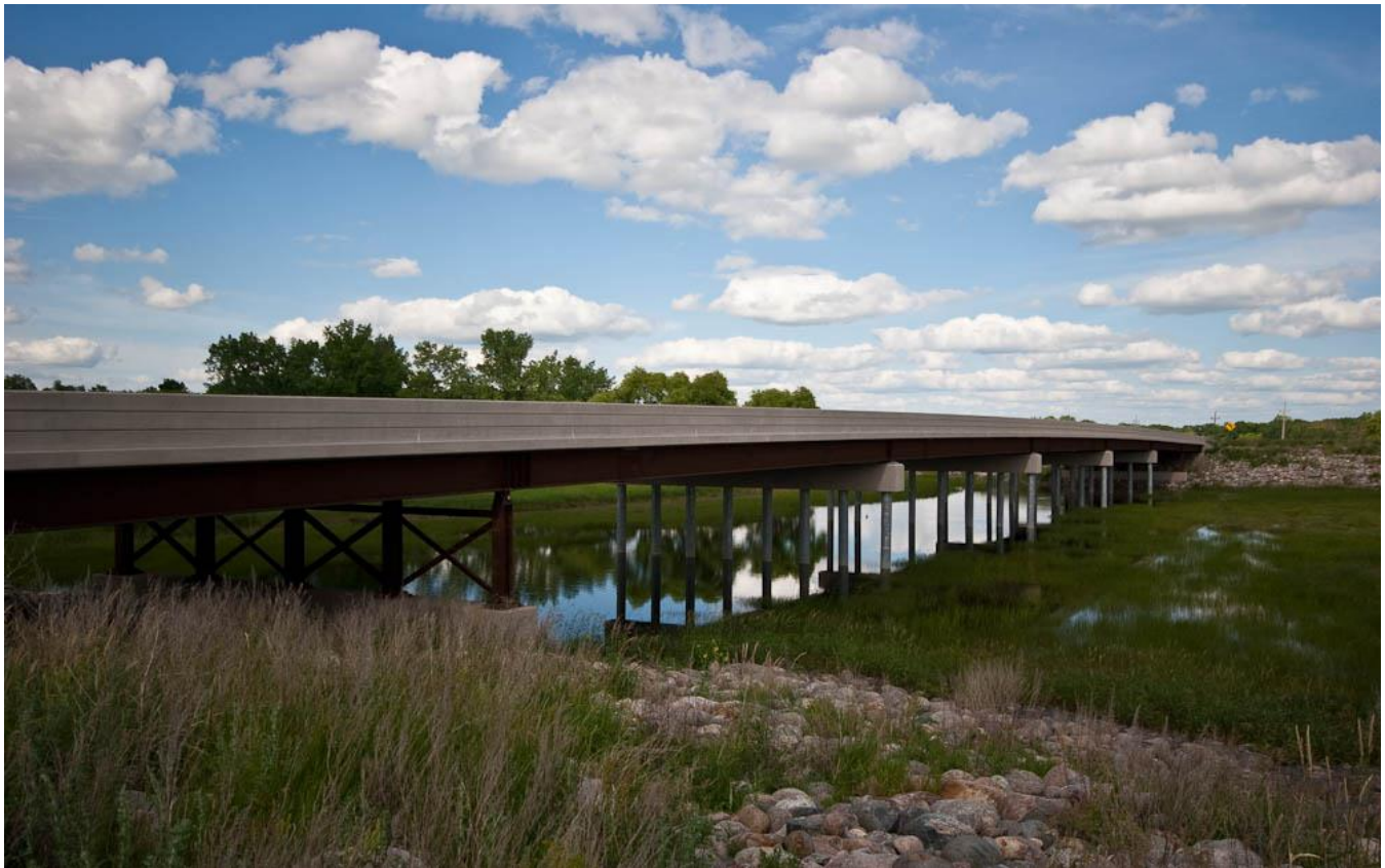
(TH171 Floodway bridge near St. Vincent, Kittson County MN)
