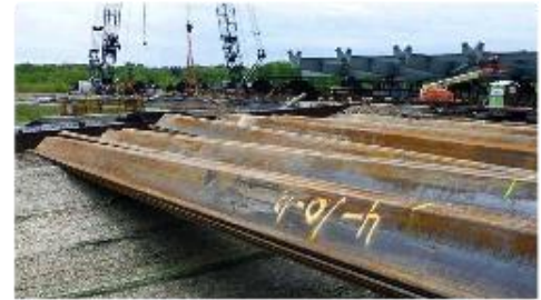
Figure 3. Drying will also kill aquatic organisms. Lay out materials to dry in the proper time. Drying times vary by species. Inspect after drying period is over. Photo credit: Dwayne Sterlund, MnDOT
