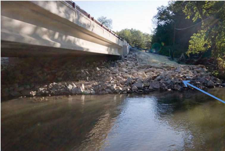
(TH30 Bucksnot Bridge, Fillmore County MN)
