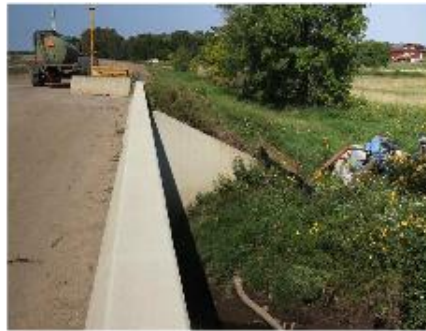
Figure 5. Pumping from designated infested waters for use elsewhere on the project is prohibited without a permit. Photo credit: Peter Leete, DNR
