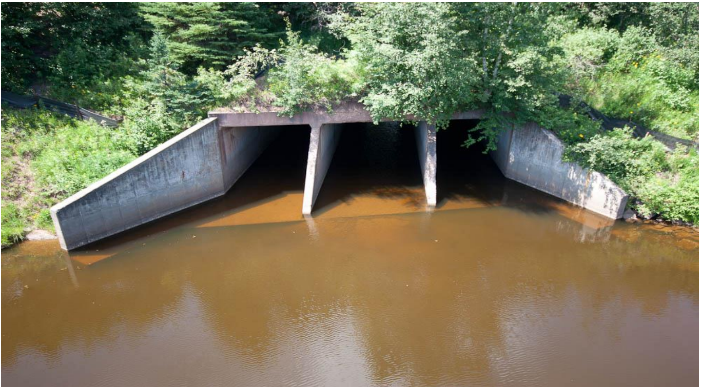
This type of flow effect is more common on low gradient streams than on high gradient streams where fully perched conditions are more likely. If the water levels drop this will create too low a depth for fish passage (TH61 Split Rock River and Lake Superior, Lake County MN).
