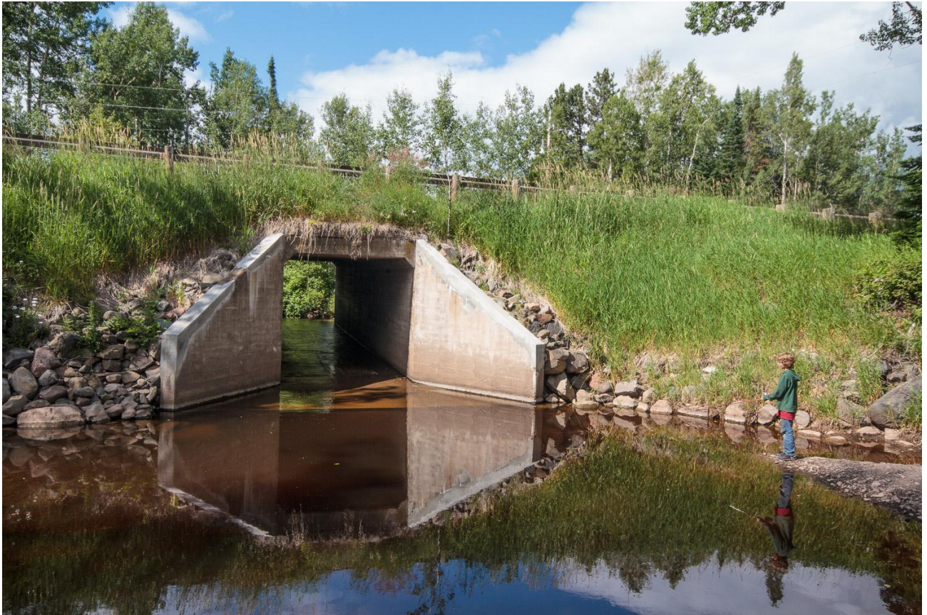
TH61 Carlson Creek at normal flow after floor overlay and grade control installation downstream (Cook County)
