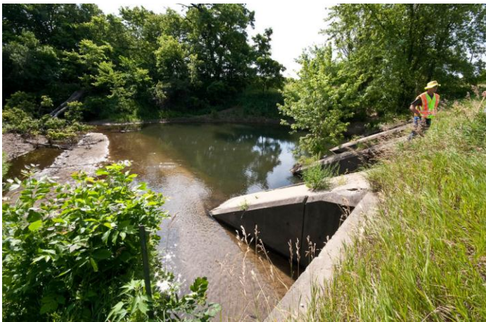
Scour holes can often be seen in air photo review. They are typical of undersized culverts and found throughout the state in a variety of topography (top left, Mississippi River, Itasca State Park, TH73, TH56, TH23)
