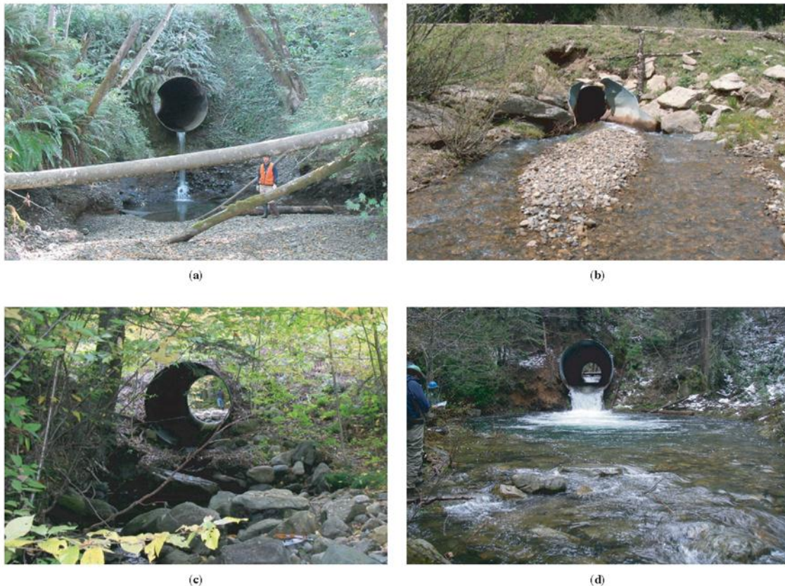
FIGURE 1 Effects of undersized culverts on channel morphology and fluvial processes: (a) upstream view of 6-ft (1.8-m) diameter culvert on Save Creek (Olympic National Forest, Washington), (b) downstream view of 3-ft (0.96-m) diameter culvert on North Thompson Creek (White River National Forest, Colorado), (c) upstream view of 6-ft (1.8-m) diameter culvert on unnamed stream (White Mountain National Forest, New Hampshire), and (d) upstream view of 9-ft (2.7-m) diameter culvert on Peavine Creek (Tahoe National Forest, California).
