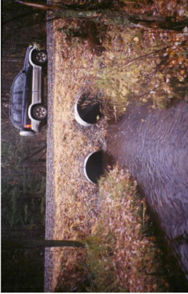
Properly sized and placed culverts.
