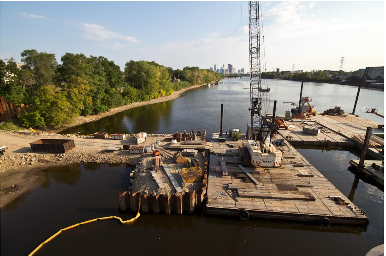
(Lowry Ave Bridge, Minneapolis, Hennepin County. photo Peter Leete)
