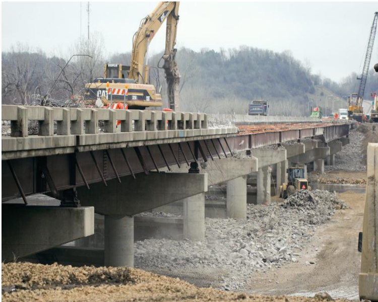
figure 1. Temporary causeway built for demolition and construction
