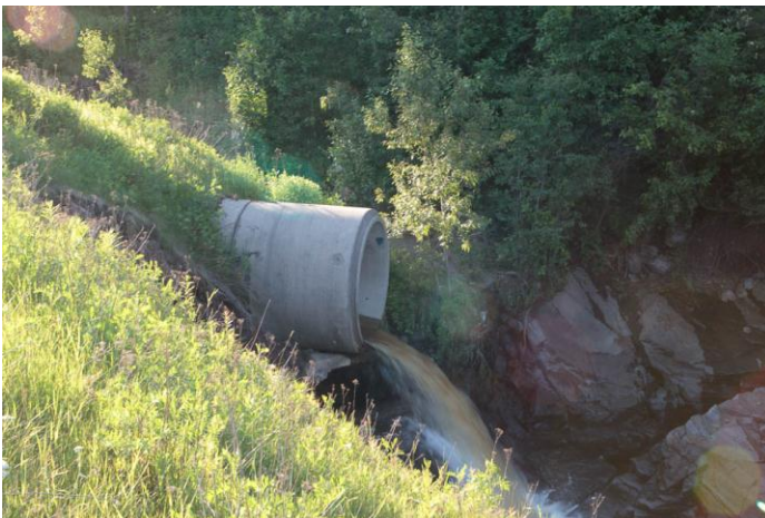
Four examples above are all along the North Shore of Lake Superior. Higher gradient streams are more prone to perched conditions, though it can happen throughout the state.
