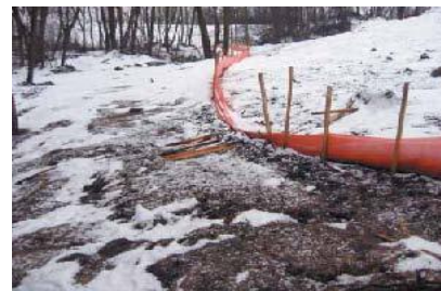
Regular maintenance is needed to ensure that a site's perimeter control is functioning properly.
