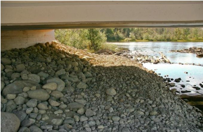
Figure 2. Bench may be constructed of any size 'walkable' aggregate
