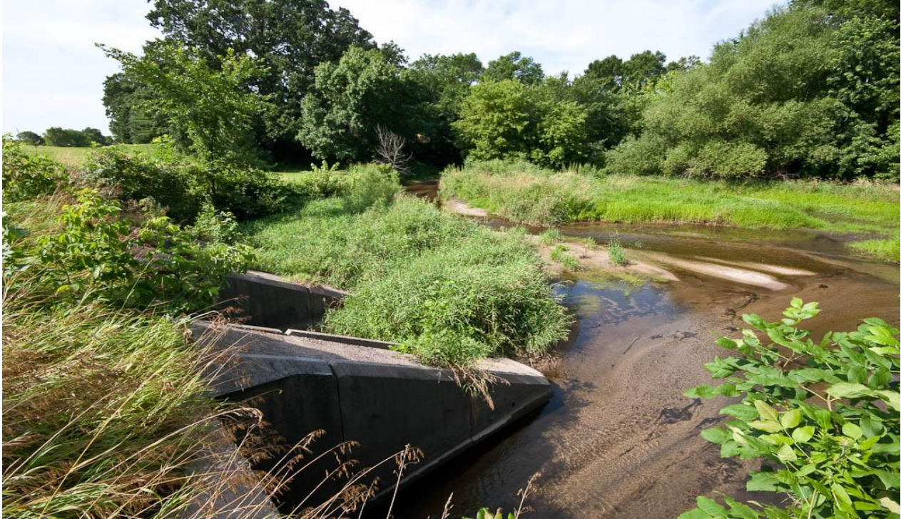
The photo above shows upstream aggradation (deposits). This area may look good, but the braided wide shallow channels through sediments is indicative of sediment deposition. Below is the downstream side of the same crossing which show the presence of a large scour hole. Having both features on the same crossing is sometimes called the 'hourglass' effect. (TH56 Freeborn County MN)
