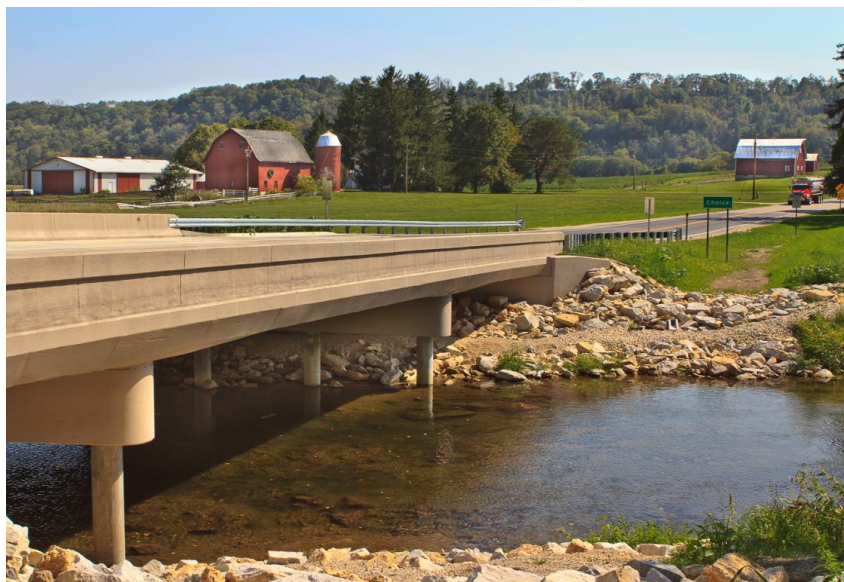
(TH43 Choice Bridge, Fillmore County)
