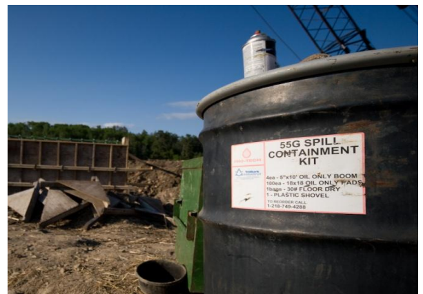
figure 7. Spill Containment kit must be on site
