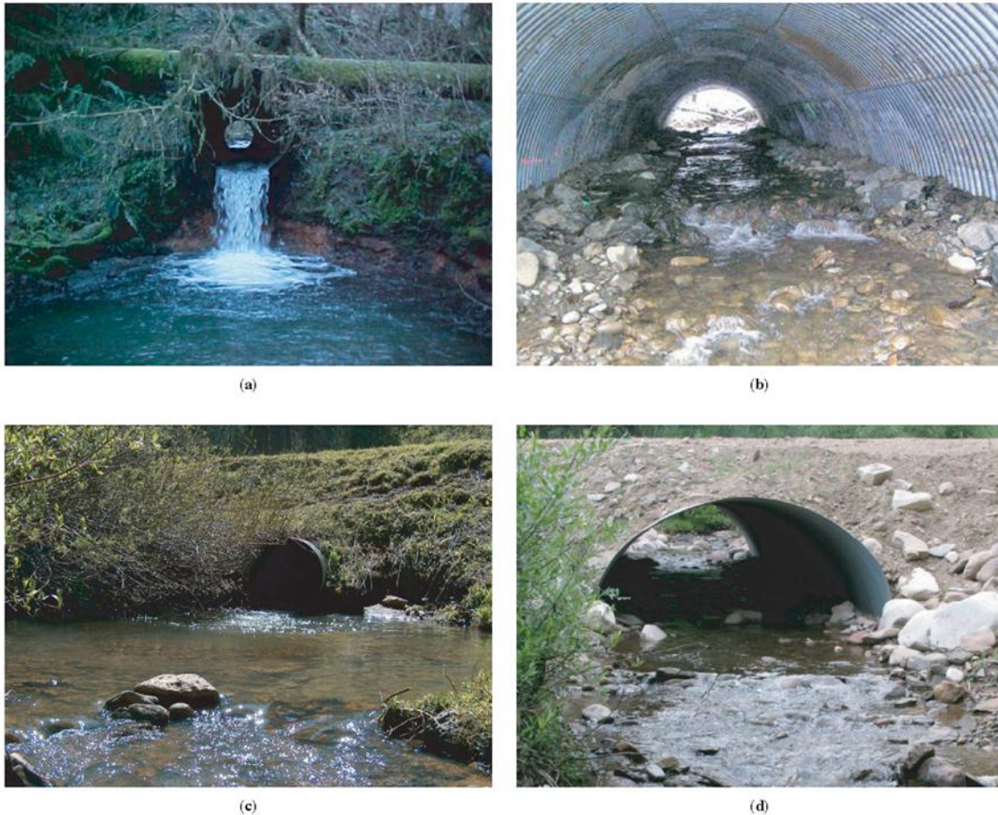
FIGURE 2 Road–stream crossings: (a) culvert built in late 1950s with diameter of 6 ft (1.83 m), length of 90 ft (27.4 m), and gradient of 2.1% before replacement along tributary to Middle Fork Salmon River, Washington; (b) same site as in (a) after the culvert was replaced using stream simulation design approach with open-bottom arch built in late 2005 with span of 18 ft (5.5 m), height of 9 ft (2.7 m), length of 95 ft (28.9 m), and gradient of 4.0%; (c) culvert built in late 1960s with diameter of 3 ft (0.96 m), length of 48 ft (14.6 m), and gradient of 2.0% before replacement along North Thompson Creek, Colorado; and (d) same site as in (c) after culvert was replaced using stream simulation design approach with pipe-arch culvert built in late 2008 with span of 12.2 ft (3.7 m), height of 8.5 ft (2.6 m), length of 48 ft (14.6 m), and gradient of 2.5%.
