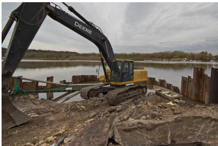
Coffer dams made of sheet metal to isolate the work area from the surface water.
