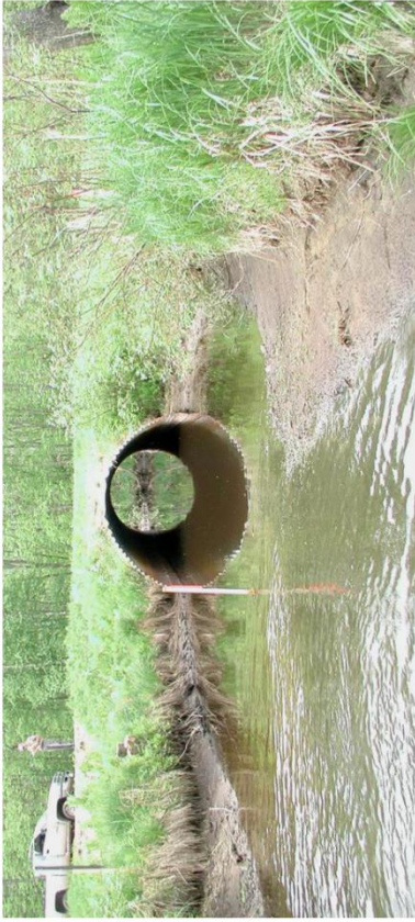
Undersized culvert.
