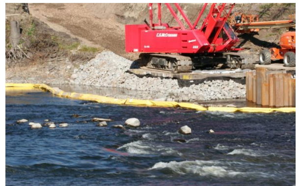
figure 6. Access pad with filter fabric pad and silt curtain for waterway protection.
