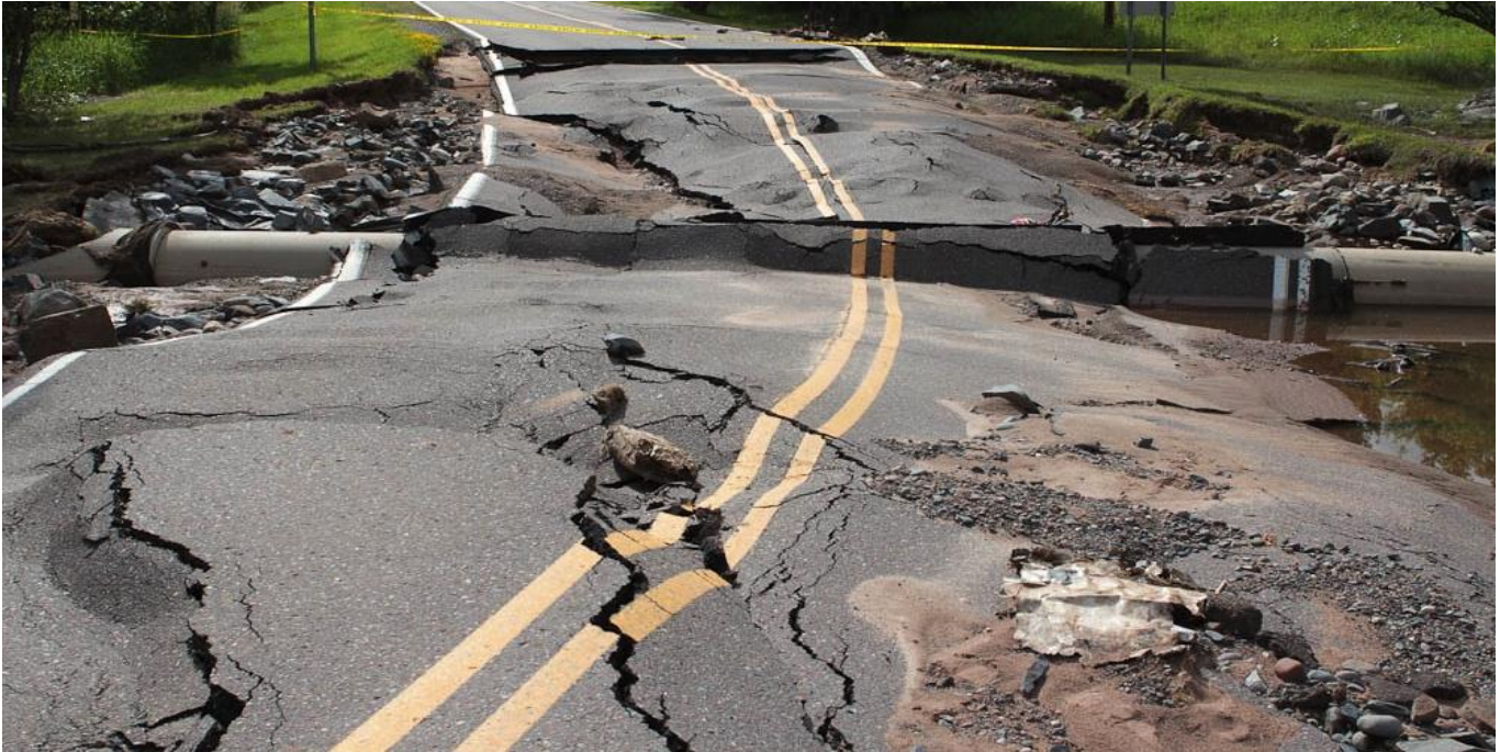
Extreme example, though valid for pointing out what can happen with overtopping. (TH210, City of Thompson, Carlton County MN)
