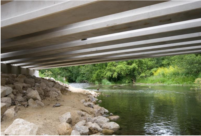
Figure 1. Completed Passage Bench
