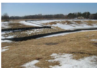
Silt fence used as perimeter control
