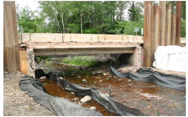
figure 4. Redundant BMPs for added protection of the waterway
