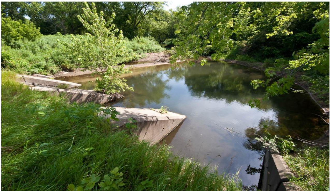
The photo above shows upstream aggradation (deposits). This area may look good, but the braided wide shallow channels through sediments is indicative of sediment deposition. Below is the downstream side of the same crossing which show the presence of a large scour hole. Having both features on the same crossing is sometimes called the 'hourglass' effect. (TH56 Freeborn County MN)
