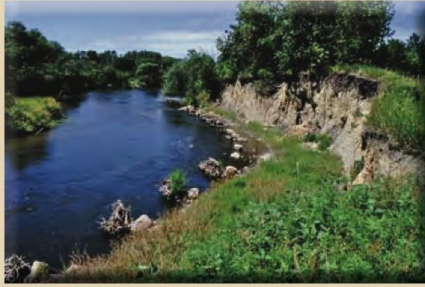
Root wad revetment and a revegetated bankfull bench built to stabilize a cutbank encroaching on Interstate 94, two years after construction (looking downstream).
