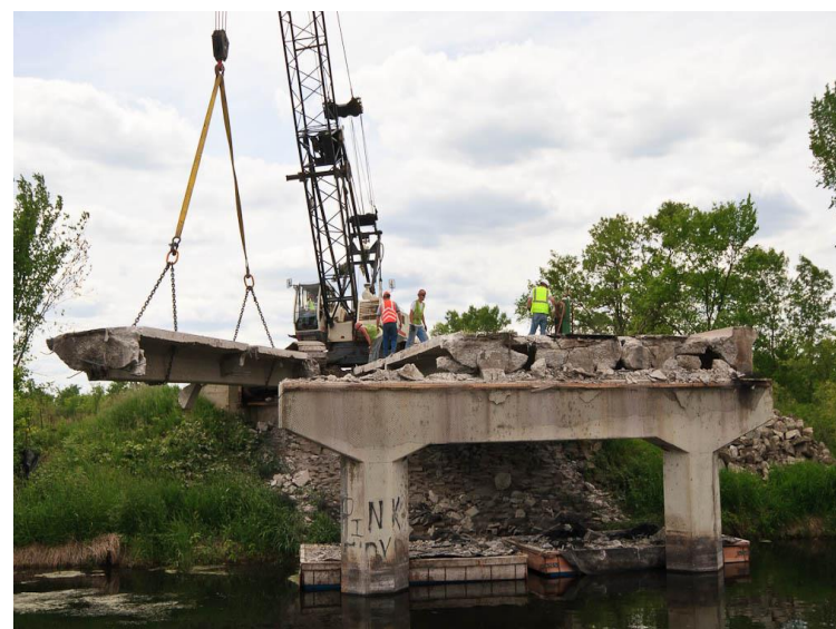
figure 3. Cut and lifting sections instead of dropping debris
