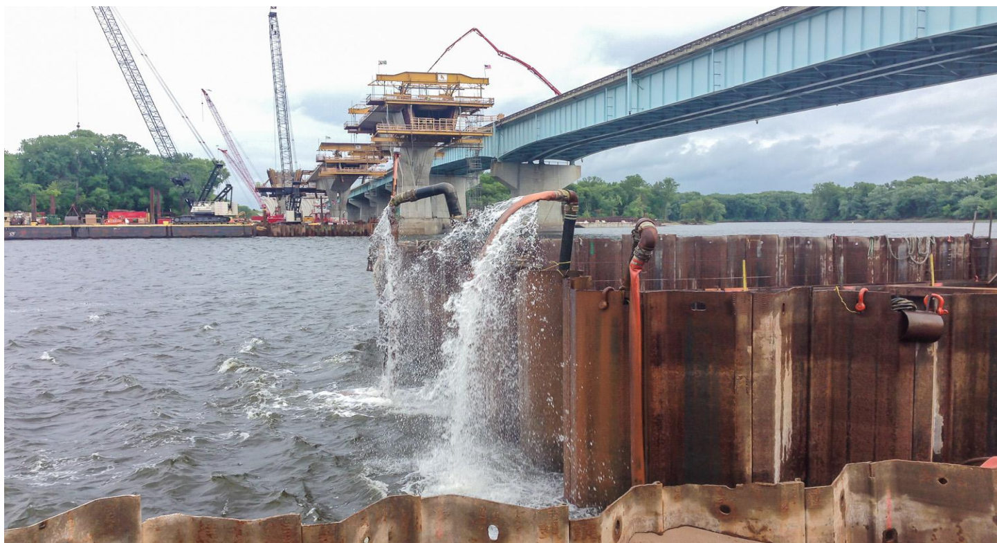
I-90 Mississippi River Bridge Replacement, Dresbach, MN
