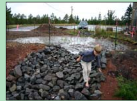
After: a rain garden is planted to treat stormwater runoff
