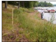
Lake shore stabilization site
