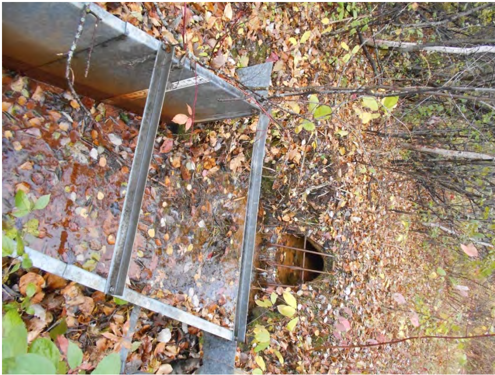
Photo 17 Outlet to monitoring flume – Looking East
