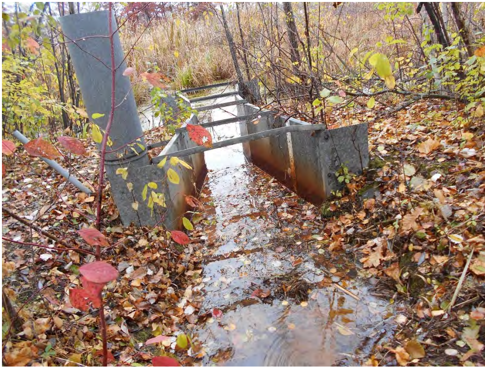
Photo 15 Monitoring flume south of potential intake location – Looking West
