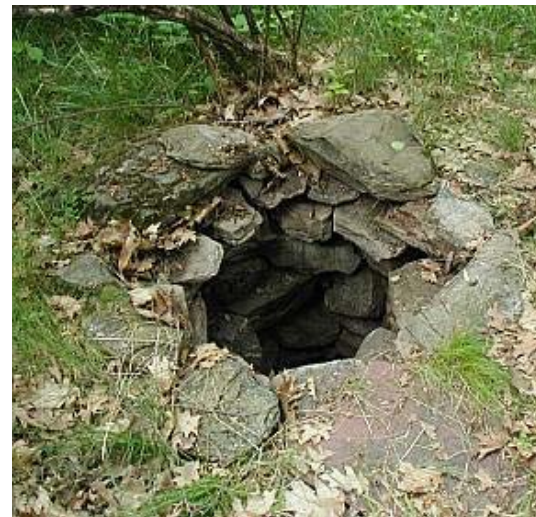
Figure 3. An uncovered dug well on an abandoned farmstead. Lined by stone, bricks, or concrete, well holes can be 3 feet to 10 feet in diameter and excavated below the water table. A dug well without a cover presents a hazard for humans and animals and a water contamination risk.
