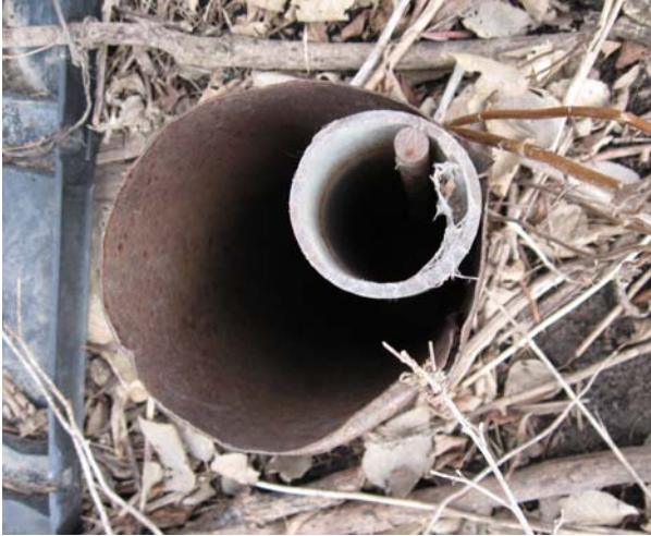
Figure 2. Looking down from above at the well casings and pump rod that have to be removed from the well before the well is sealed against contaminants.
