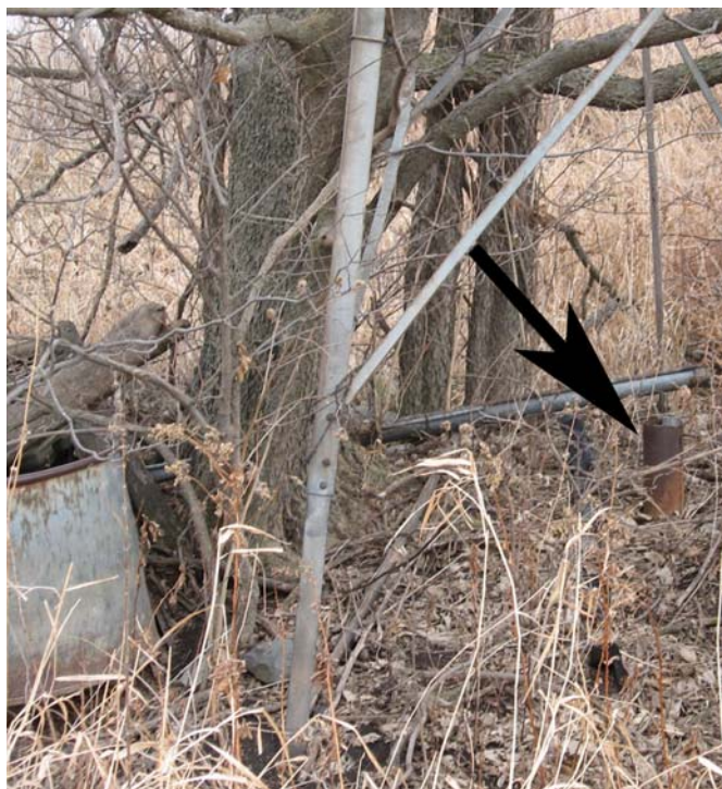
Figure 1. The windmill and open, rusty well casing (shown the by arrow) mark this abandoned well. This is a potential access point for contaminants.
