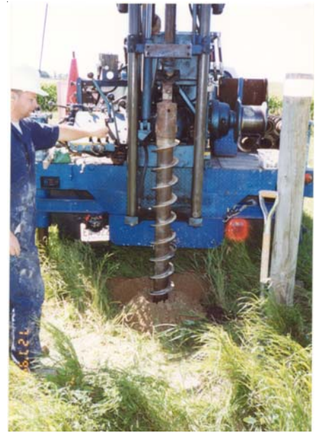
FIGURE 2. Drilling ground-water-level monitoring wells is an important step in monitoring ground-water levels in aquifers.
