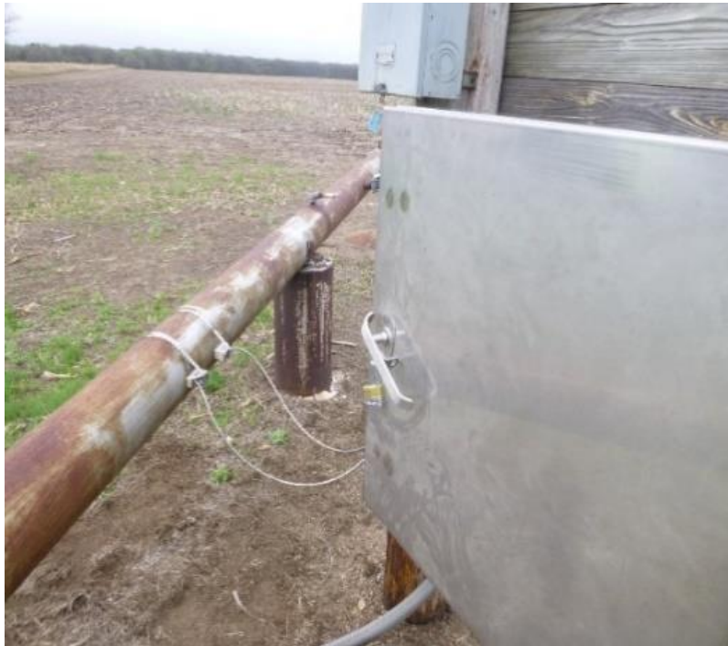
Figure 2 – Flow meter clamped to exterior of pipe
