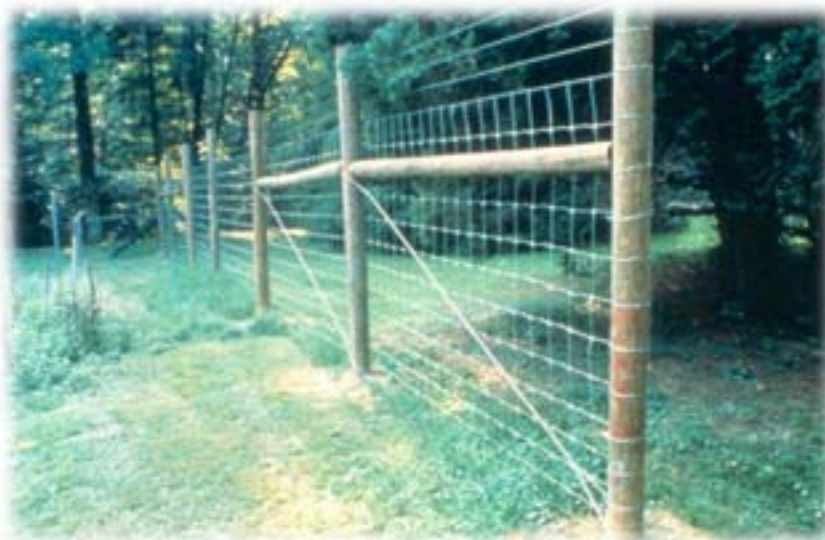
Figure 5. Double brace assembly
