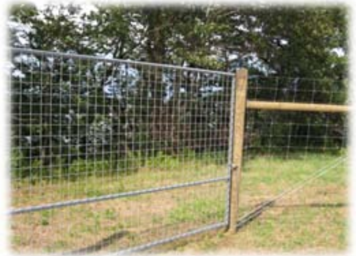
Figure 15. Two examples of custom gates available through fence supply vendors. The gate to the left is built with a stainless steel frame covered in the same fabric as the fence. The gate to the right is built with a galvanized frame and galvanized welded wire.
