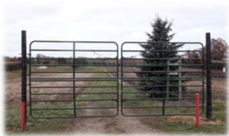
Figure 12. Four 10 ft. gate panels used for a 20 ft. opening, two for each panel.
