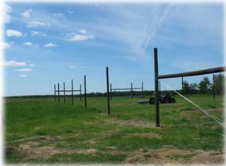
Figure 7. A small hay yard ready for the woven wire installation.
