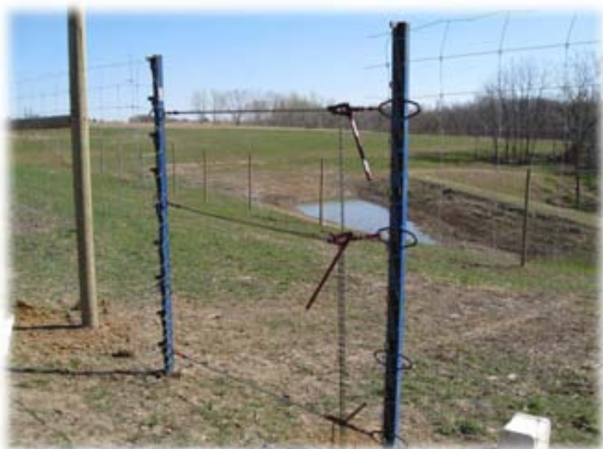
Figure 9. In the above photos the wire is pinned, using the silver wedges, to the blue stretching bars and is drawn tight with the red mechanical chain pullers.
