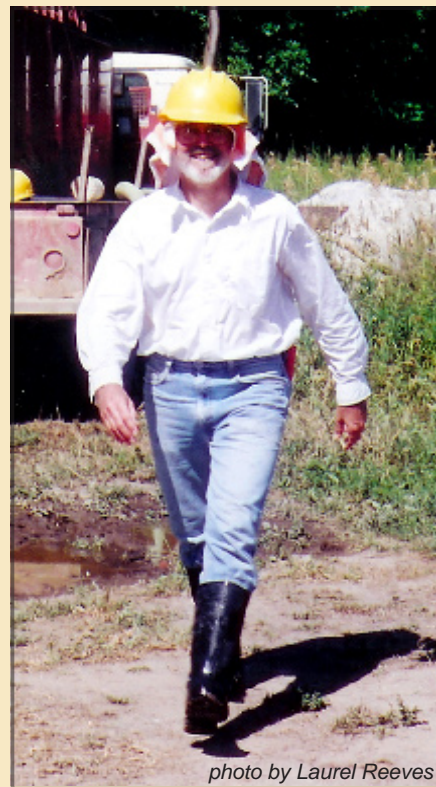
On site obwell drilling
