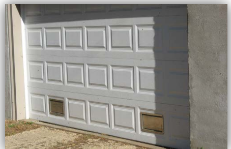
Figure 5 (below): Example of a structure with automatic openings (engineered version), which must be located on at least two sides of the structure to allow floodwaters to pass through.
