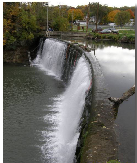
Lanesboro Dam in Fillmore Co.
