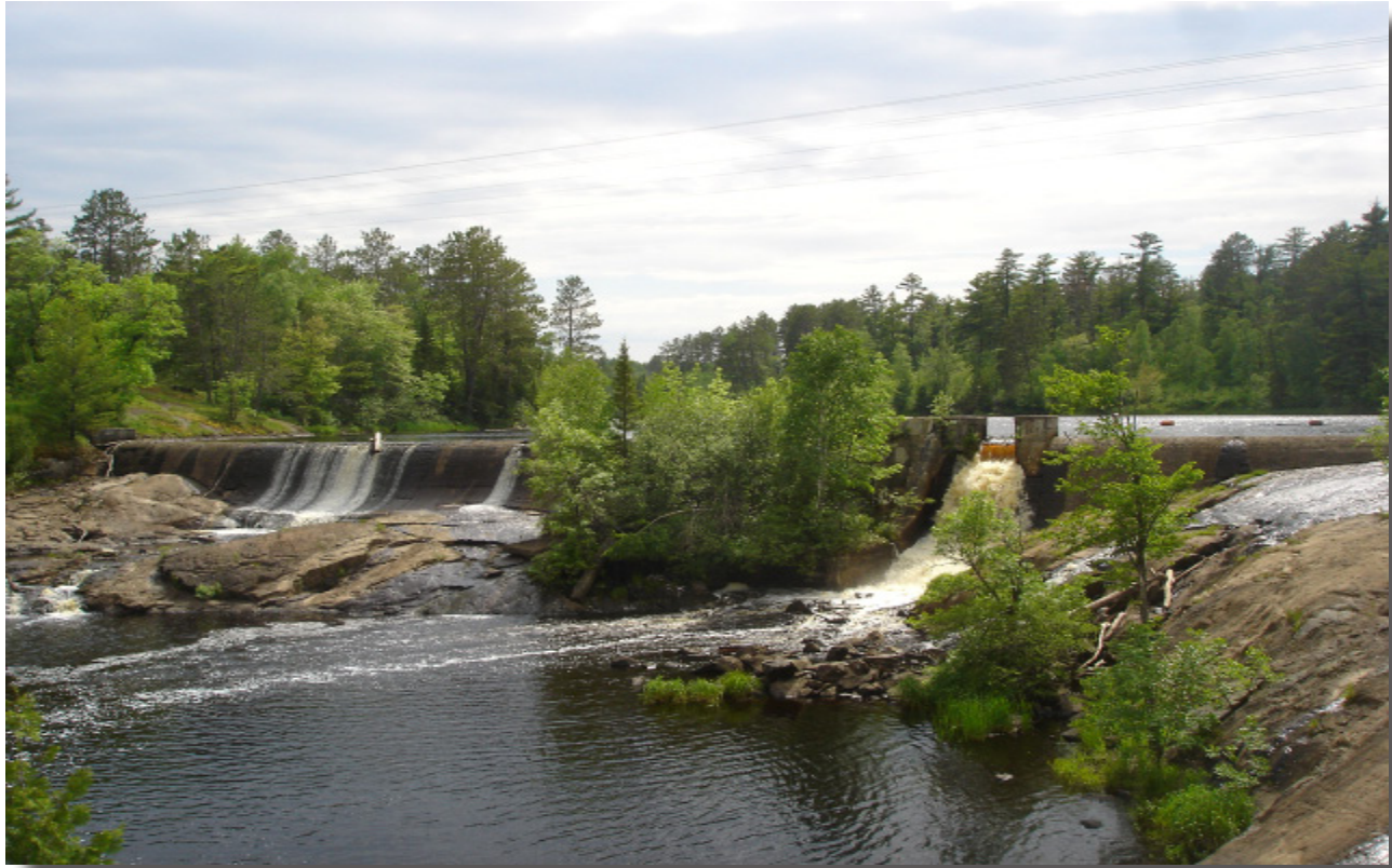
Pike River Dam in St. Louis County
