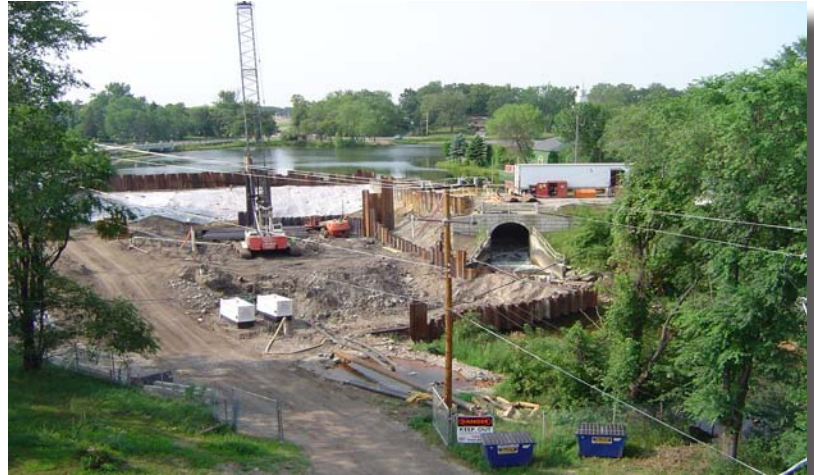
New London Dam reconstruction in Kandiyohi Co.
