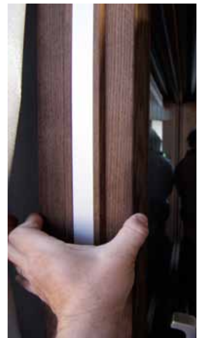
Thermally heat treated wood used in a window frame.
