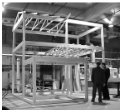
Demonstration house built at NRRI to demonstrate metal fastener and other housing fabrication technology
