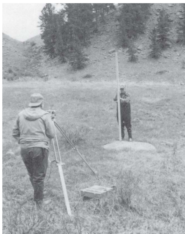
Figure 34. Shooting the elevation of the benchmark.
