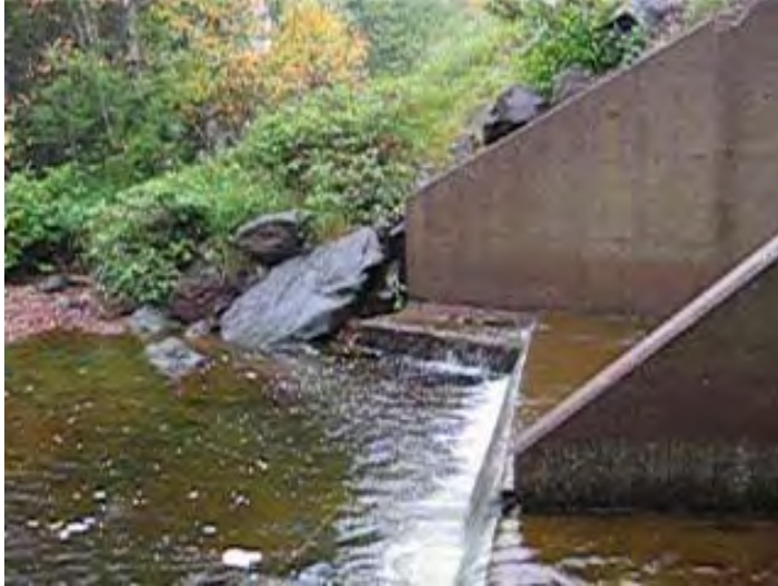
Figure 10.2. Perched culvert at the Devil Track River Highway 61 road crossing.
