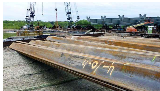
Figure 3. Drying will also kill aquatic organisms. Lay out materials to dry in the proper time. Drying times vary by species. Inspect after drying period is over. Photo credit: Dwayne Stenlund, MnDOT
