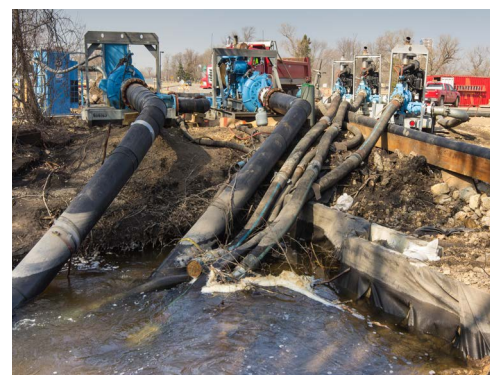
Figure 6. Drain all water from equipment where water may be trapped. Remove drain plugs and drain hoses prior to transport. Photo Credit: Peter Leete, DNR
