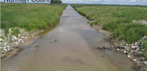
This ditched stream is filling up with sediment because it cannot move the material downstream. Note the uniformity of habitat. South Branch of the Wild Rice River, Norman County.
