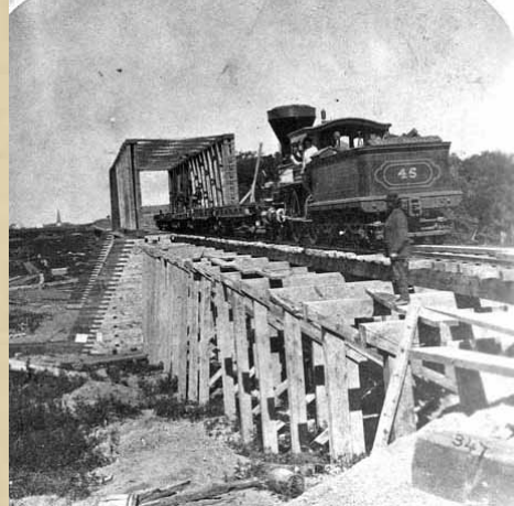
Northern Pacific work train at Fargo-Moorhead constructing first railroad bridge into Dakota Territory, 1872.
