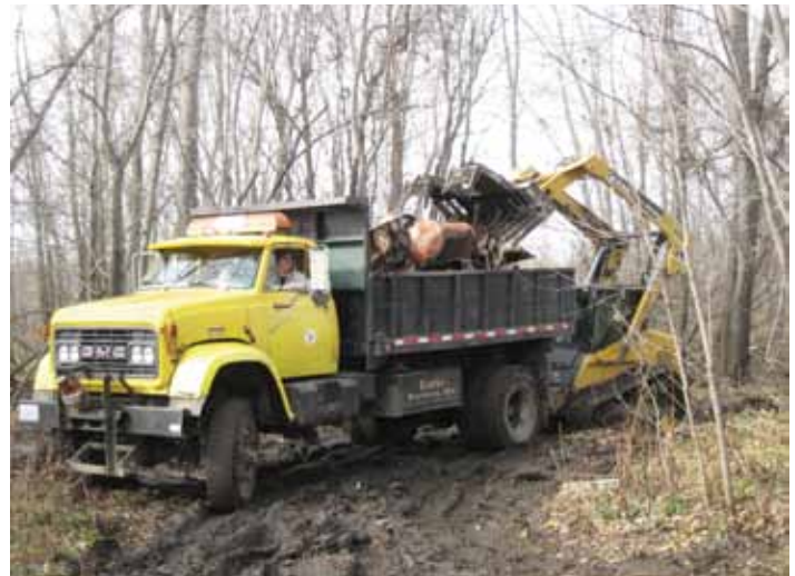
Heavy machinery from MN4WDA was used to pick up large items in the woods including tires, tanks, barrels and auto parts.
