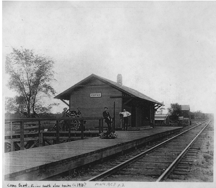
Copas Station, Copas (ca. 1910) (Minnesota Historical Society Photographic Collections Location No. MW4.9 CP p2 and Negative No. 22107).
