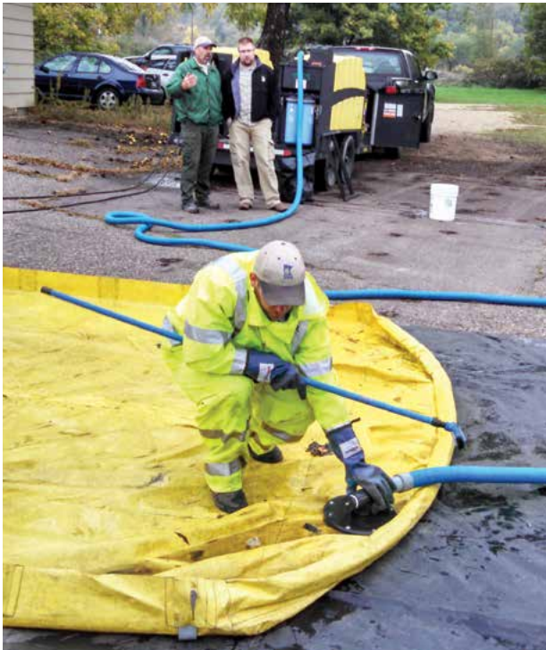
Inspector reclaims water from mat using the vacuum head attached to vacuum hose.
