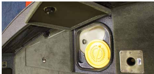
Check all water-holding compartments, like this bait well, to ensure they have fully drained.
