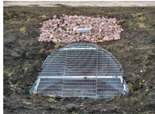
A culvert screen installed in southwestern Minnesota to prevent invasive carp moving from the Missouri River water shed into the Des Moines River watershed during high water events.
