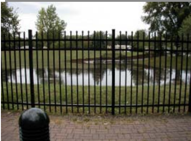
Dry storage pond after an hour of heavy rain
