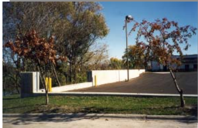
A small invisible floodwall protects downtown Breckenridge
