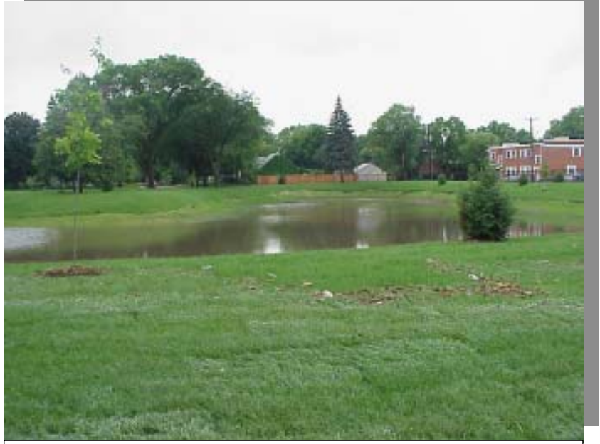
Wet storage pond at 60th & 1st Ave. in Minneapolis
