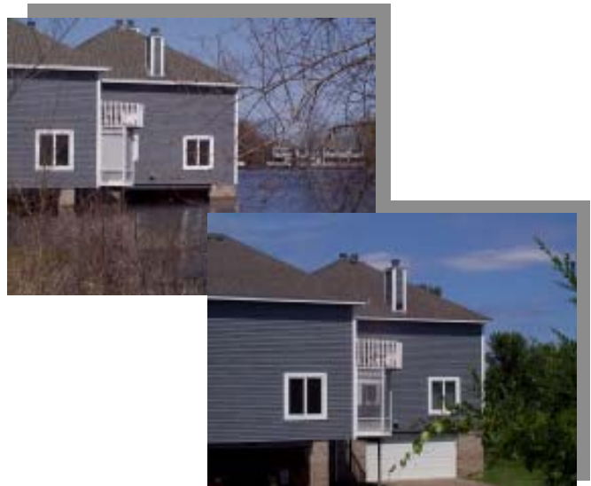
Townhouse with tuck-under garage that opens during the flood
