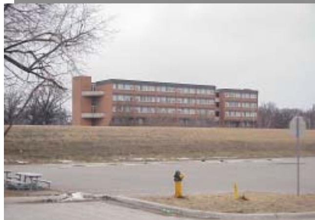
Large levee in front of Sunshine Terrace
