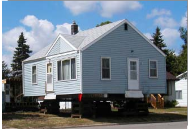
House being moved out of the floodplain in Breckenridge
