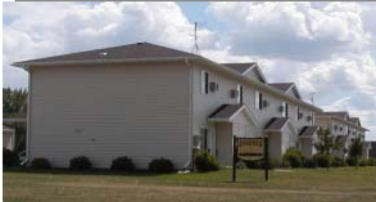
New housing units constructed after the 1997 flood
