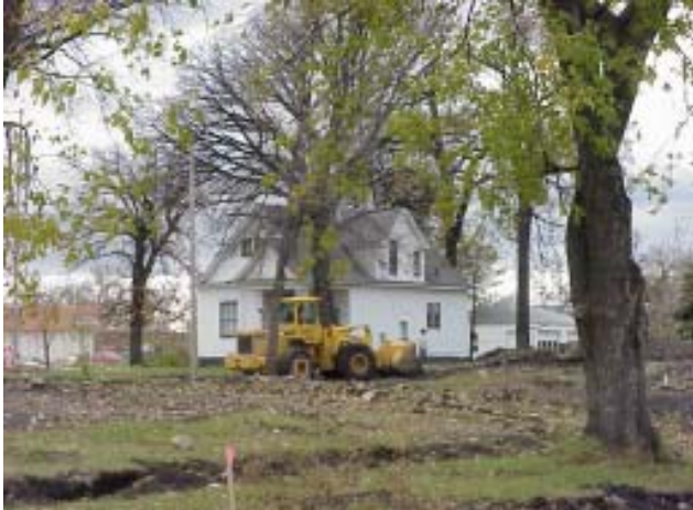
Moving damaged homes out of the floodplain
