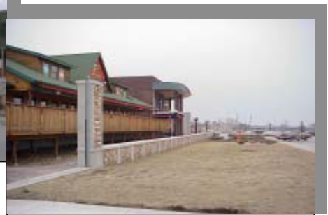
Floodwall in place
