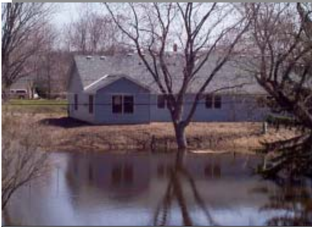
House on fill in Bayport
