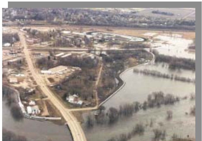
Corps will improve this levee along Gravel Road
