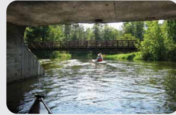
Be alert for box culverts and low culverts at the beginning of this water trail.
