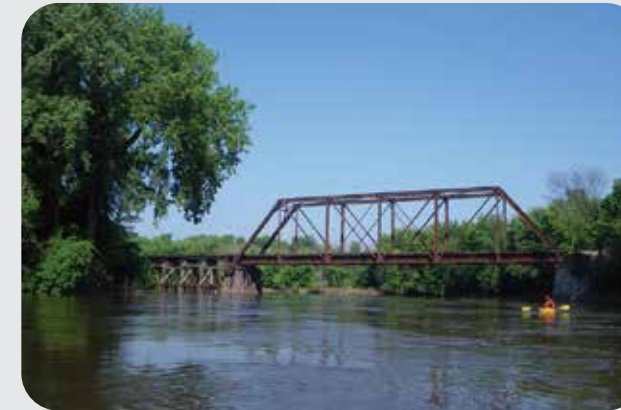
Railroad bridge at Morton.
