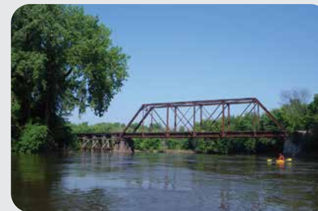
Railroad bridge at Morton.
