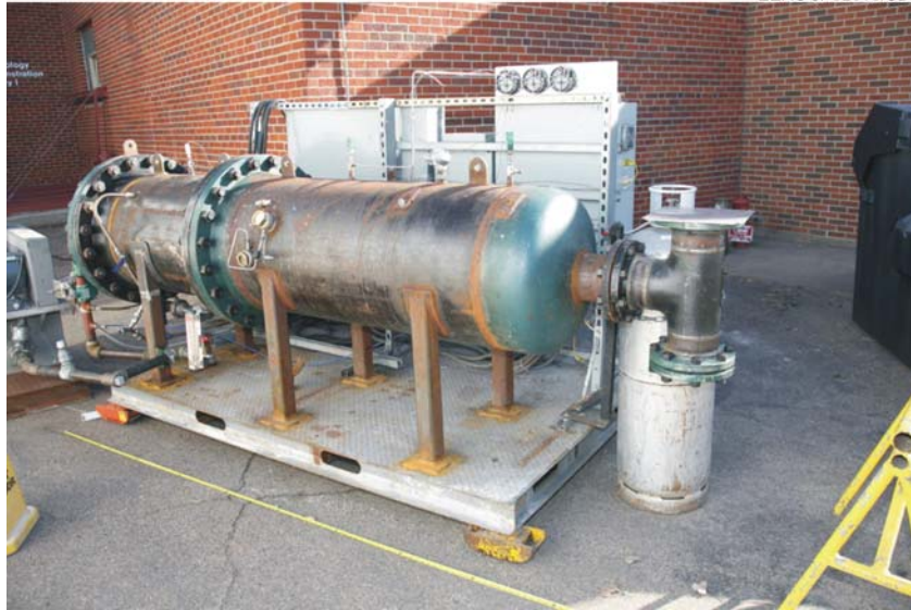
Figure 3. EERC HEDT field unit.
