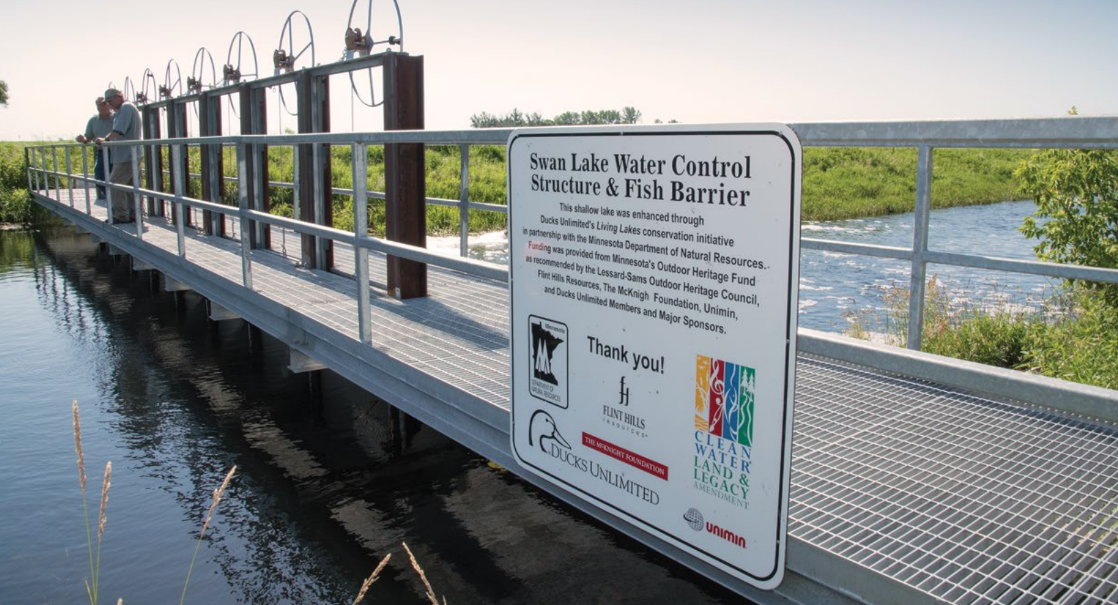
▲ Swan Lake water control structure and fish barrier. LAM staff collaborate with local governments and nonprofit conservation organizations to advance the DNR mission.
