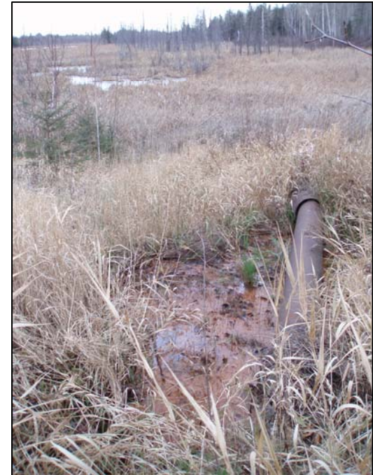
Surface seep on the north edge of Cell 2E/1E.
