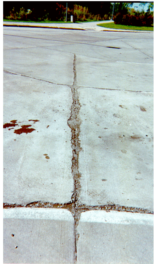
Cracked concrete Source: Mn/DOT
