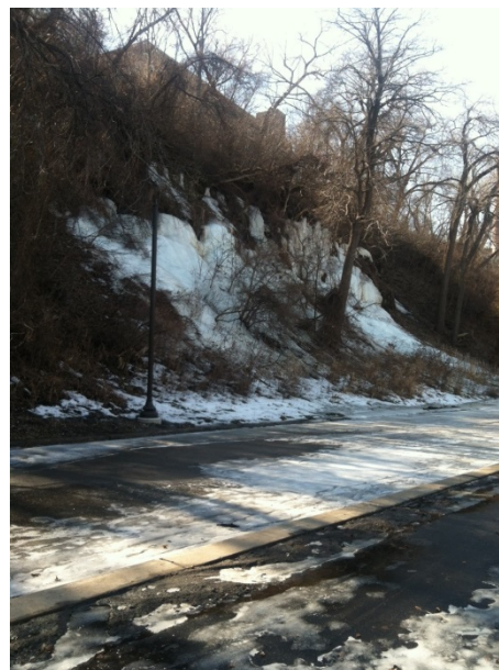
Figure 2. These icicles form at “the weeping wall” and emerge from beds within the Platteville Limestone. This photo was taken just down-river from the 2014 Fairview Hospital landslide in Minneapolis. Photo by Carrie Jennings.
