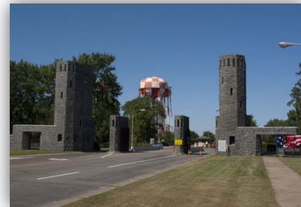
Camp Ripley entrance walls and gate
