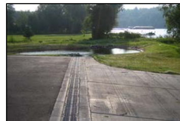
Water access rehabilitation needs include demonstrating best management practices for stormwater runoff. This site uses a slot drain for water conveyance to an infiltration basin, preventing runoff from directly draining into the lake.
