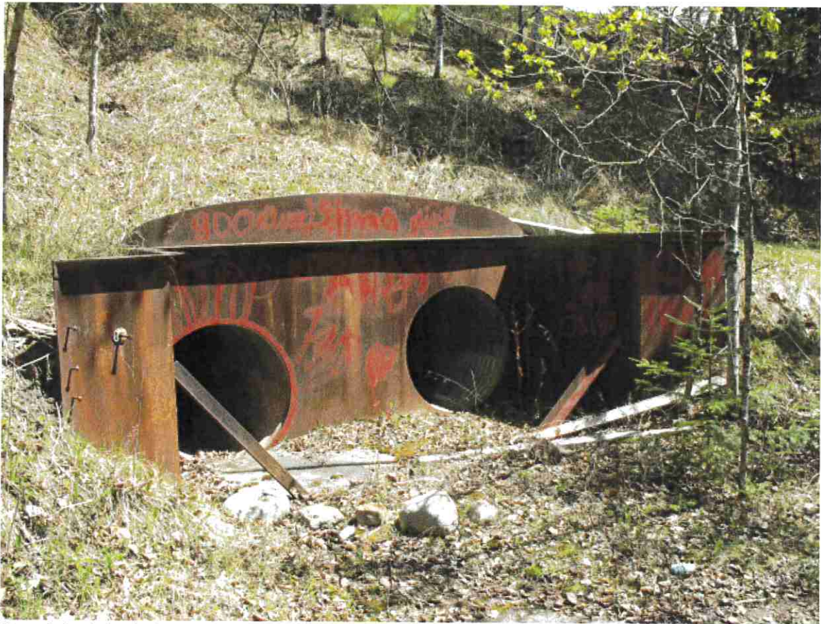
Figure 8. Steel-plated culvert abutment, photo by T. Tumberg.
