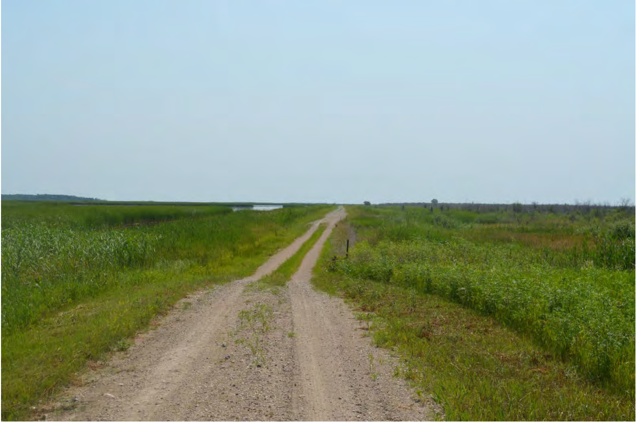
Figure 4. Picture of emergency spillway area along the south embankment of Pool 3 of the Roseau River Wildlife Management Area.
