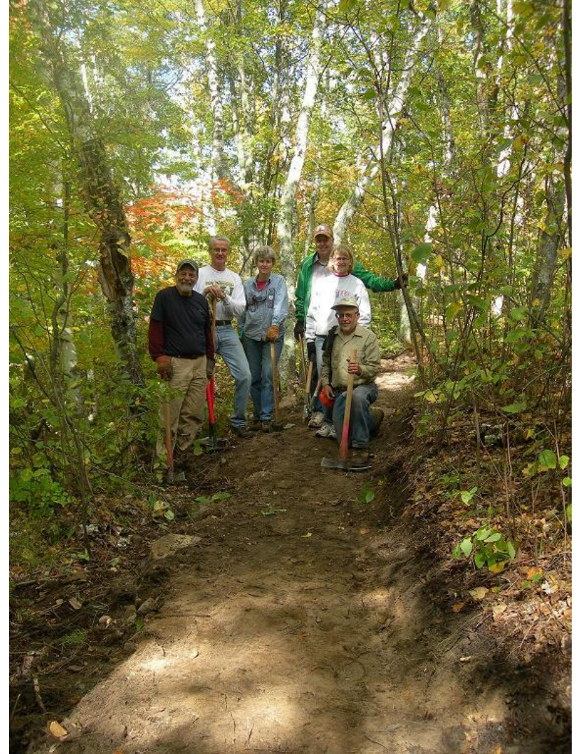
Figure 6.2 -- Side-hill Trail Construction.
