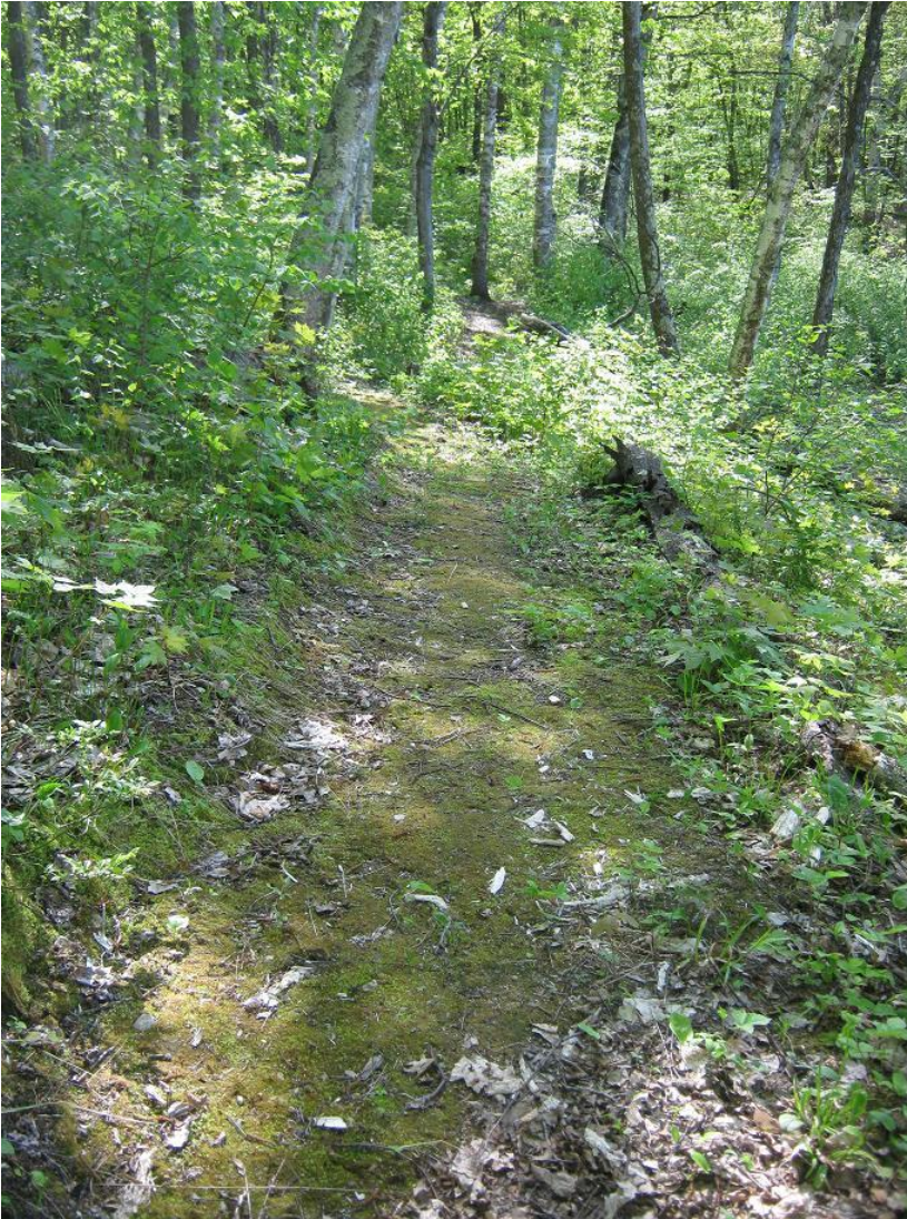
Figure 6.3 -- Treadway Stabilized by Mosses and Outsloping.
