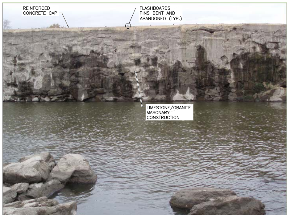
2 PHOTO: PRIMARY SPILLWAY (2006 DRAWDOWN) C-07 NOT TO SCALE
