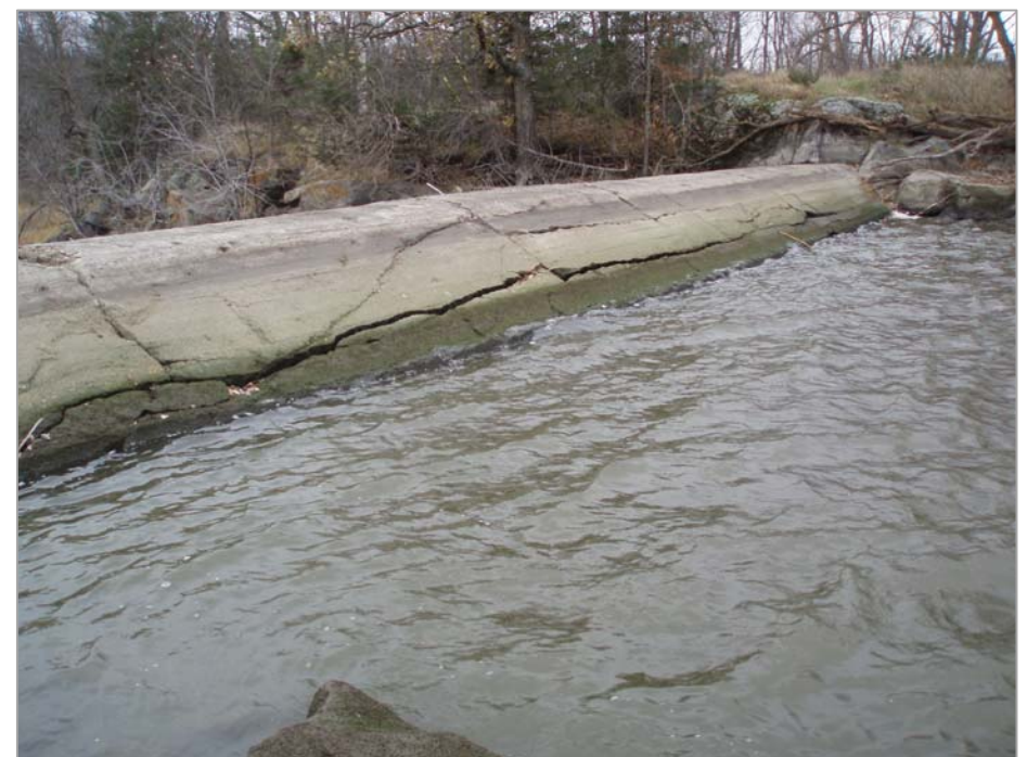
6 PHOTO: SECONDARY SPILLWAY (2006 DRAWDOWN) C-07 NOT TO SCALE
