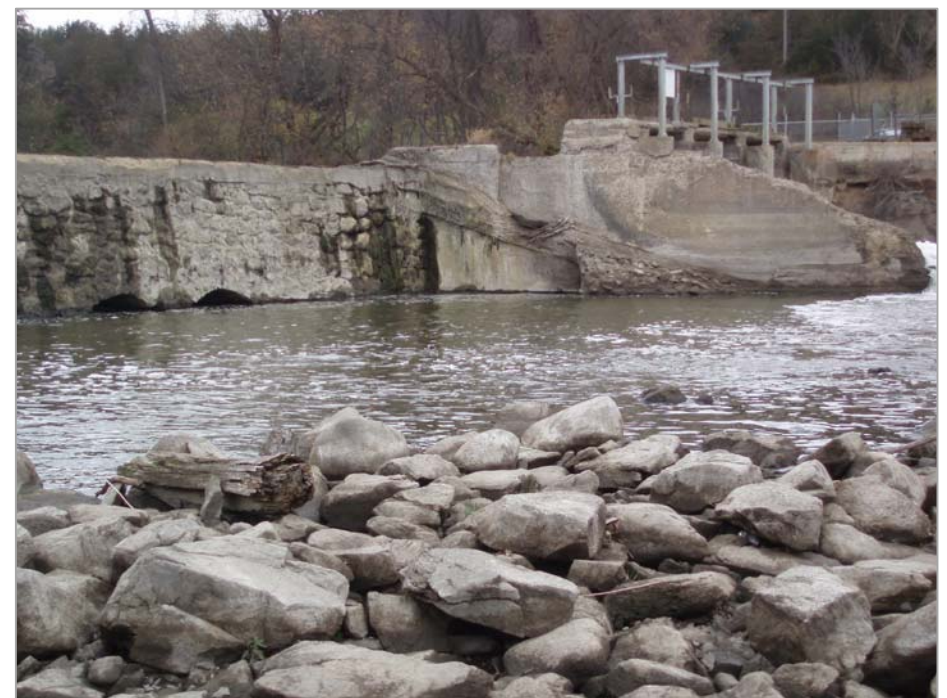
5 PHOTO: PRIMARY SPILLWAY AND SPILLWAY/STOPLOG ABUTMENT (2006 DRAWDOWN) C-07 NOT TO SCALE
