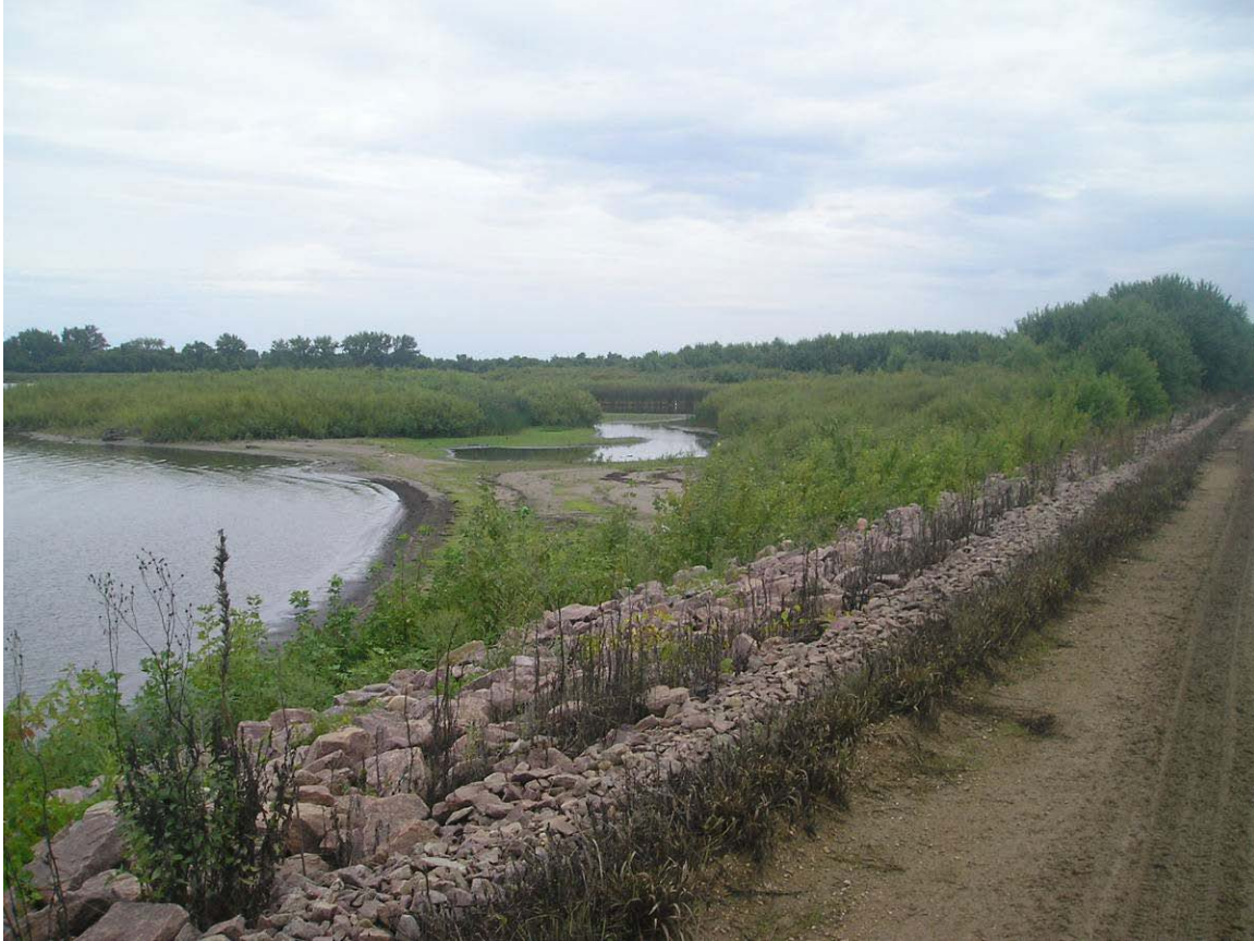
Figure 2-8. Pomme de Terre River delta where it enters Marsh Lake. Looking north from the Marsh Lake Dam.
