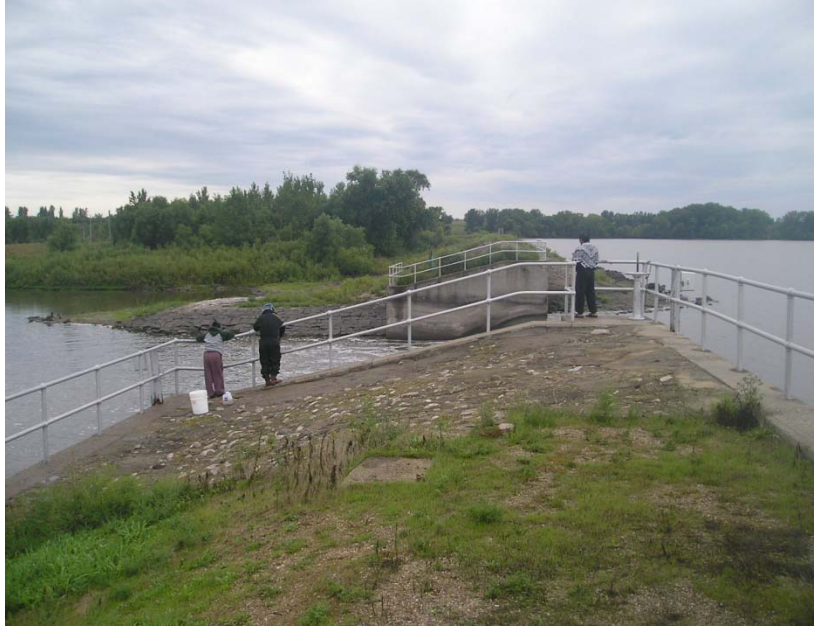
Figure 7-1. Existing Marsh Lake spillway looking south.
