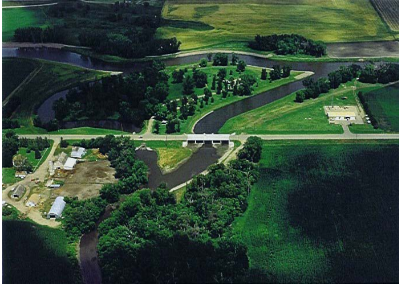
Figure 1-5. Chippewa River Diversion on the Chippewa River near Watson, Minnesota. Diversion structure is under bridge at center, Watson Sag Channel at upper left.
