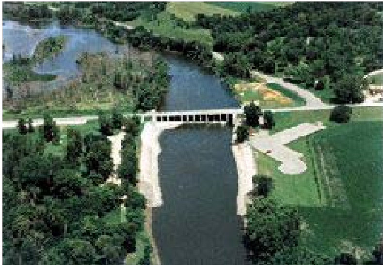
Figure 1-4. Lac qui Parle Dam on the Minnesota River, looking upstream.
