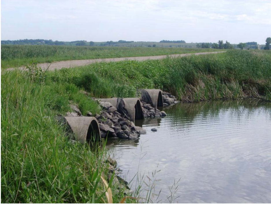
Figure 4-9. Culverts under the Louisburg Grade Road at the upper end of Marsh Lake.
