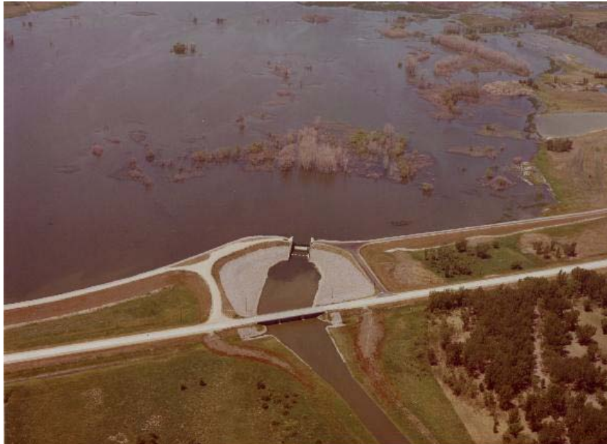
Figure 1-7. Highway 75 Dam on the Minnesota River.
