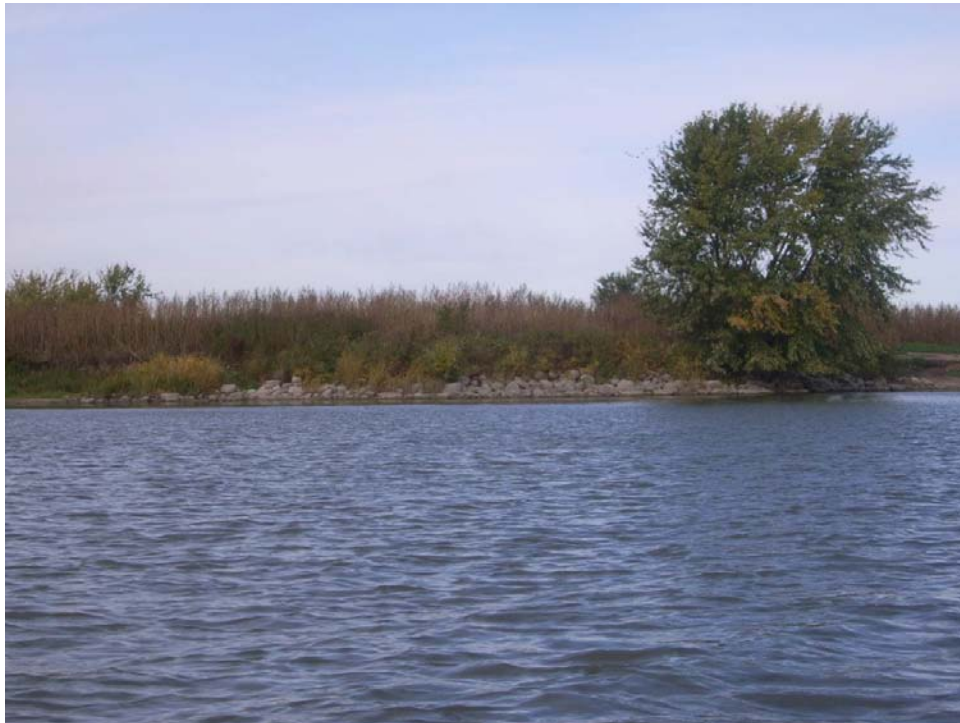
Figure 2-13. Eroding shoreline on an island in Marsh Lake armored by native boulders. October 9, 2008 photo.
