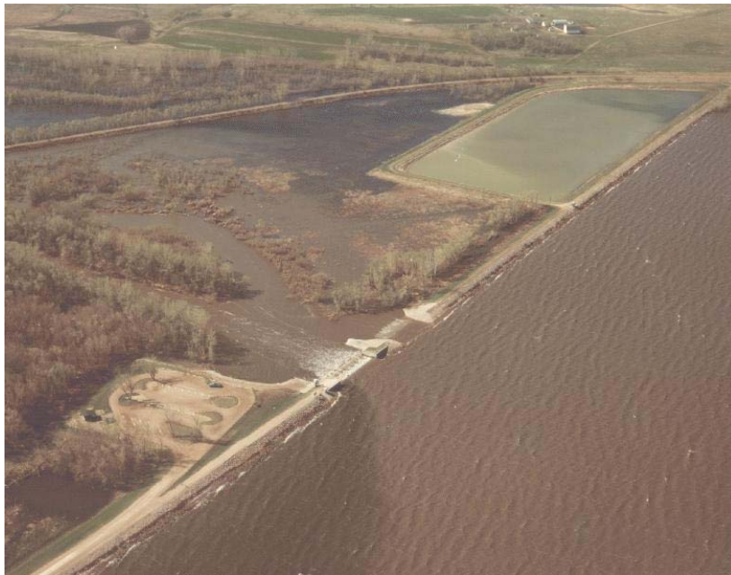
Figure 1-6. Marsh Lake Dam on the Minnesota River. Abandoned fish rearing pond at upper right on downstream side of dam.
