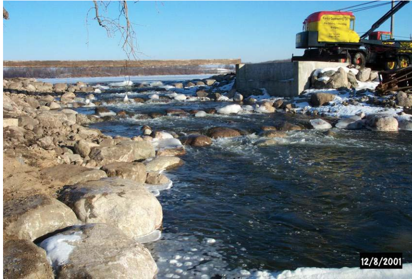
Figure 4-3. Rock ramp fishway at a lake outlet. Minnesota DNR photo.
