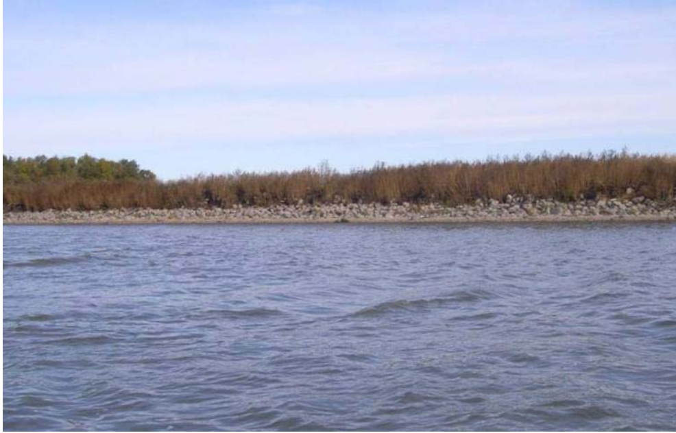
Figure 2-12. Eroding shoreline along the north side of Marsh Lake armored by native boulders. October 9, 2008 photo.
