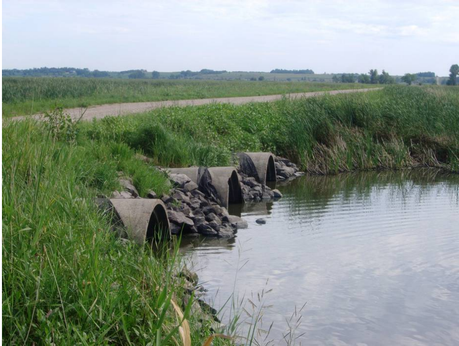
Figure 6. Existing culverts under the Louisburg Grade Road at the upper end of Marsh Lake.
