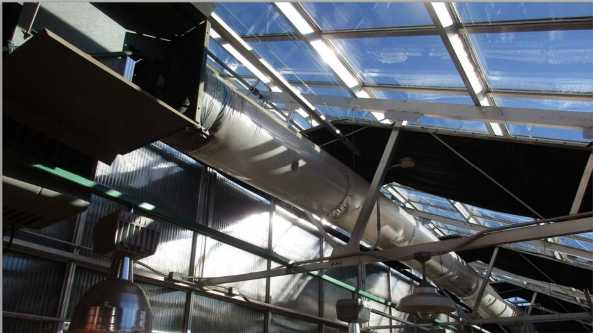
Figure 2: Greenhouse Heating Duct
