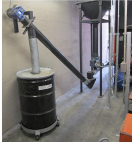
**Figure 13 – Automated Ash Collection from Pellet/Chip Boiler**
