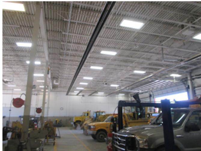
**Figure 5 – Garage Area with Overhead Radiant System**
